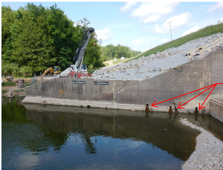
Photo 33: Right side (west) downstream retaining wall showing map cracking, large spall with exposed reinforcing steel and temporary construction railing.
