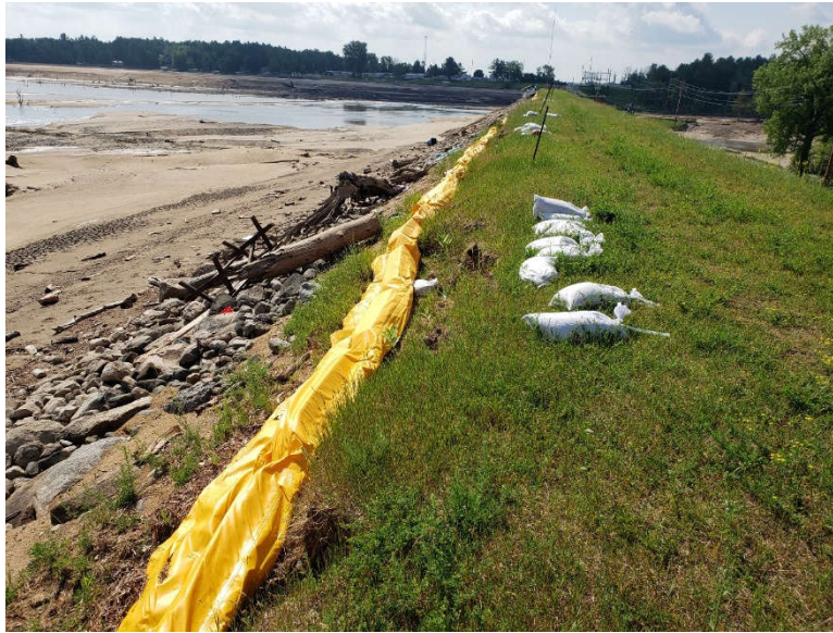
Photo 19: Upstream slope of Right Embankment – Tittabawassee. Note tension cracks that have developed at crest.
