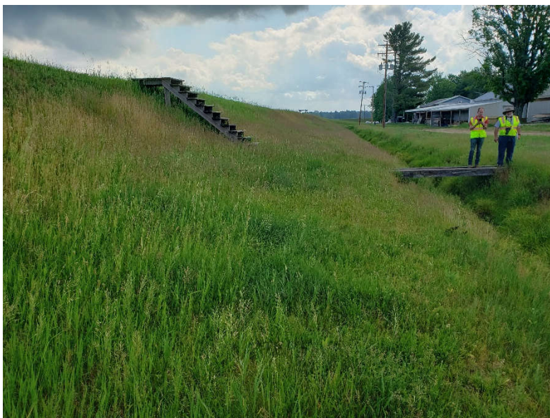
Photo 23: Downstream slope of Left Embankment – Tobacco.
