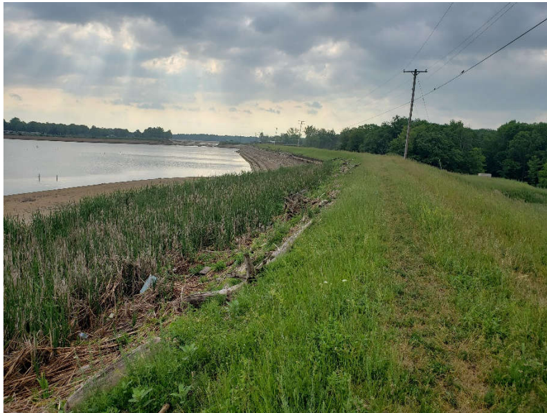
Photo 43: Upstream slope of Right Embankment – Tittabawassee that will require slope protection to be reestablished (vegetation and riprap).
