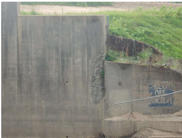
Photo 7: Left (east) side retaining wall downstream general elevation including spall with exposed rebar (6'x2'x3").
