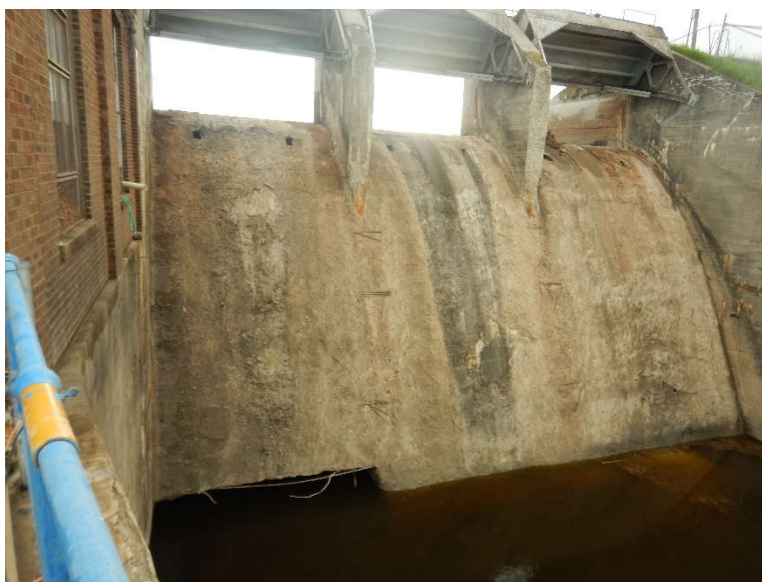
Photo 5: Spillway general elevation with extensive spalling, exposed reinforcing steel and likely delamination.
