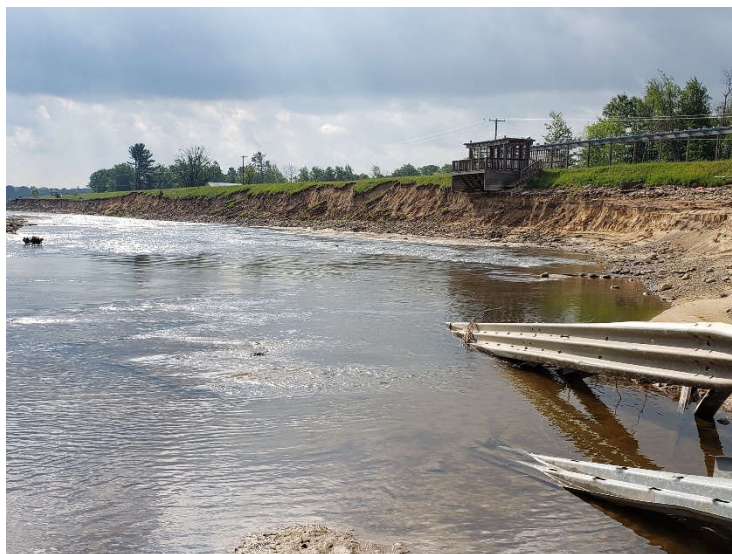
Photo 26: Upstream slope of Left Embankment – Tobacco that has been severely eroded and requires immediate protection.
