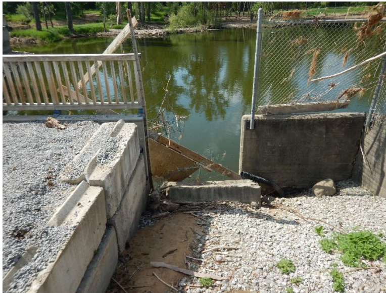
Photo 38: Left (east) side cutoff wall isolated with concrete cribbing.
