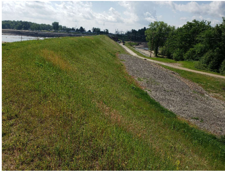
Photo 21: Downstream slope of Right Embankment – Tittabawassee.
