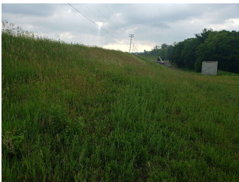
Photo 42: Downstream slope of Right Embankment – Tittabawassee. Established vegetation and minimal slope adjustment/movement and seeps present.
