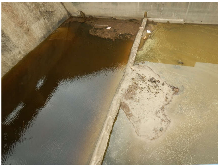
Photo 6: Weir exhibiting large spalls with exposed reinforcing steel and sediment deposits.
