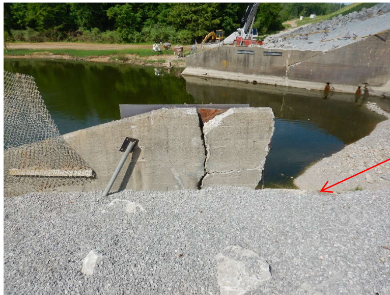
Photo 31: Back face of left side (east) retaining wall at steel reinforcing plate. Notice horizontal cut just right of plate.
