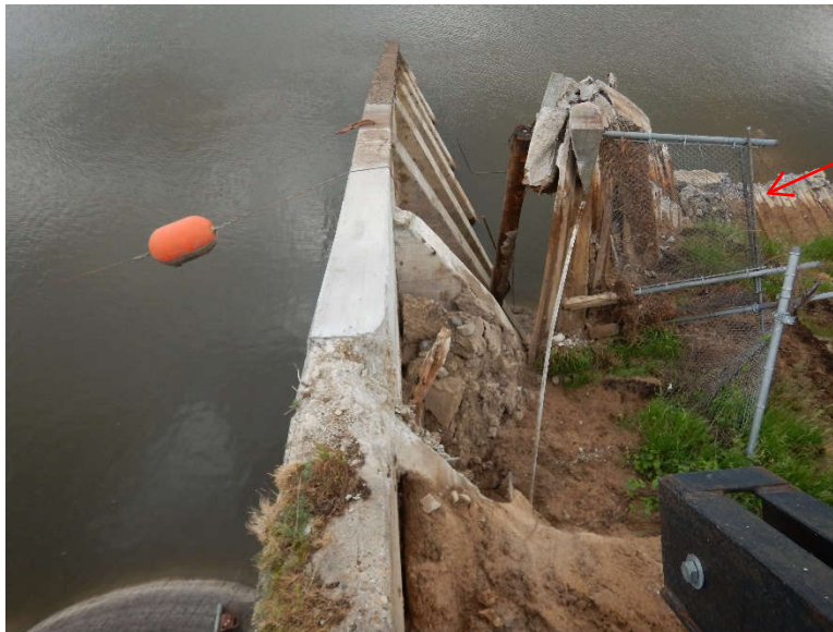
Photo 12: Erosion behind left side (east) retaining wall at upstream end.
