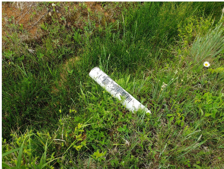
Photo 44: Toe drain outlets not discharging at time of inspection.
