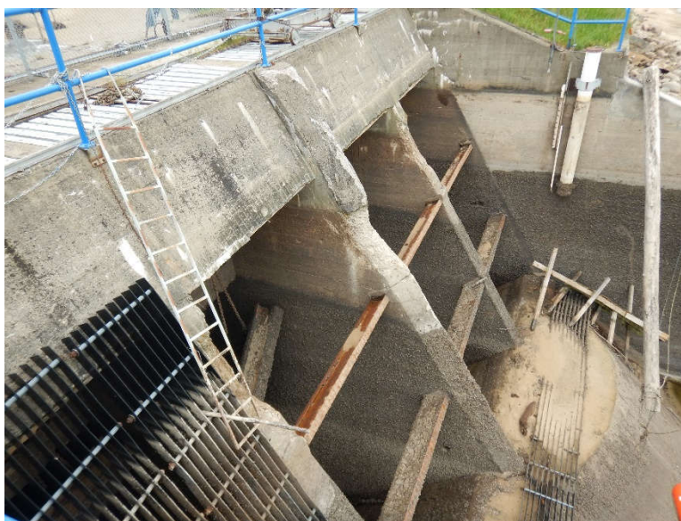
Photo 16: Powerhouse intake piers with spalls and displaced or missing trash racks.
