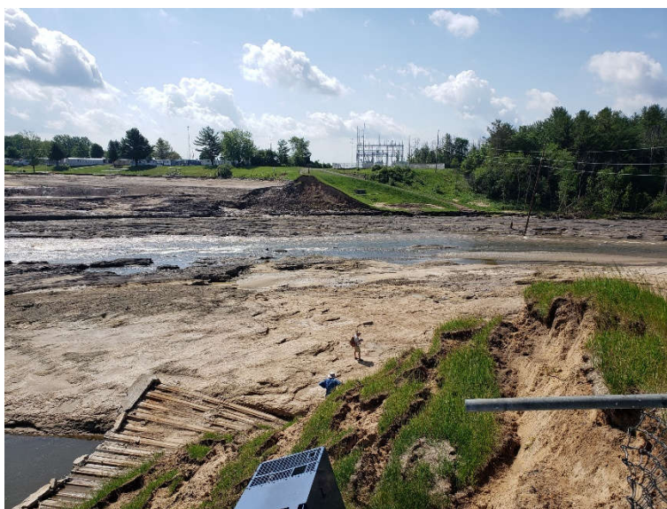
Photo 1: Breached section of the Left Embankment – Tittabawassee section looking left.
