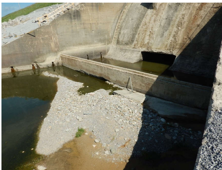
Photo 29: Tobacco spillway weir with large spall and sediment.
