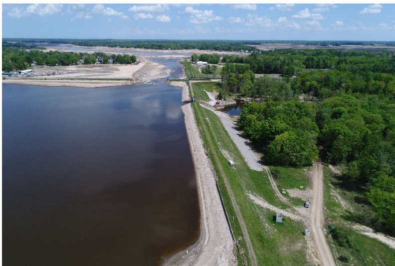
Photo 41: Overall view of Right Embankment – Tittabawassee (drone photo provided by EGLE).
