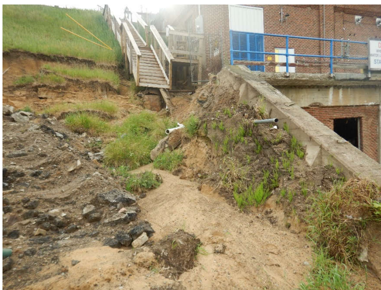
Photo 10: Erosion behind right side (west) retaining wall at downstream end.
