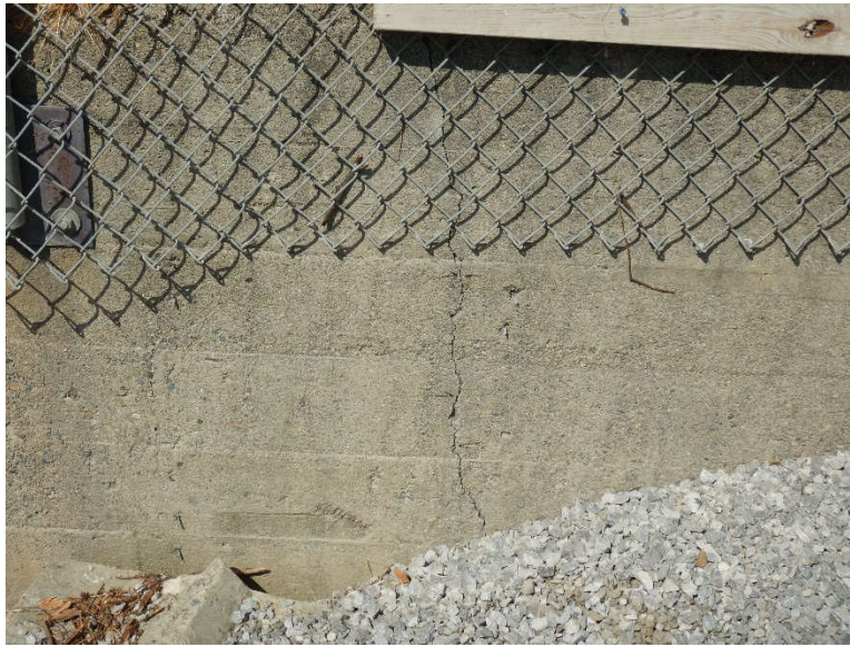
Photo 32: Vertical crack on back face of left side (east) retaining wall near downstream end.
