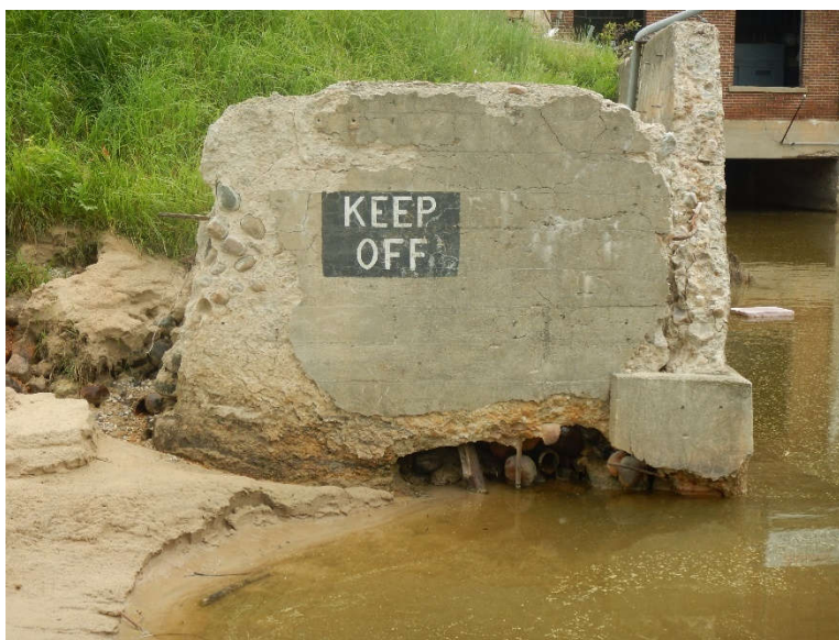
Photo 14: Right side (west) cutoff wall with large spalls/hole with exposed reinforcing steel.
