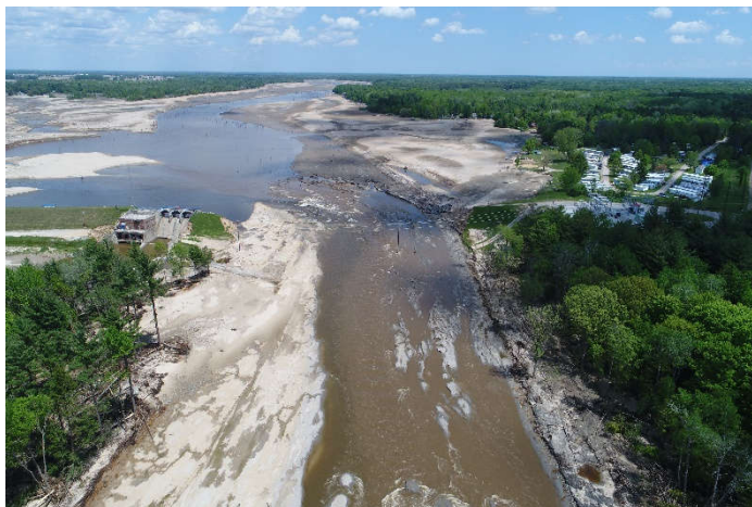
Photo 3: Breached section of embankment where drainage is currently cutting in a new alignment (drone photo provided by EGLE).
