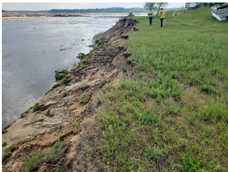
Photo 25: Upstream slope of Left Embankment – Tobacco that has been severely eroded and requires immediate protection.
