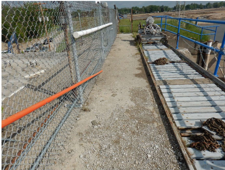
Photo 4: Typical condition of deck looking east. Note recently painted safety railings and deterioration of concrete.
