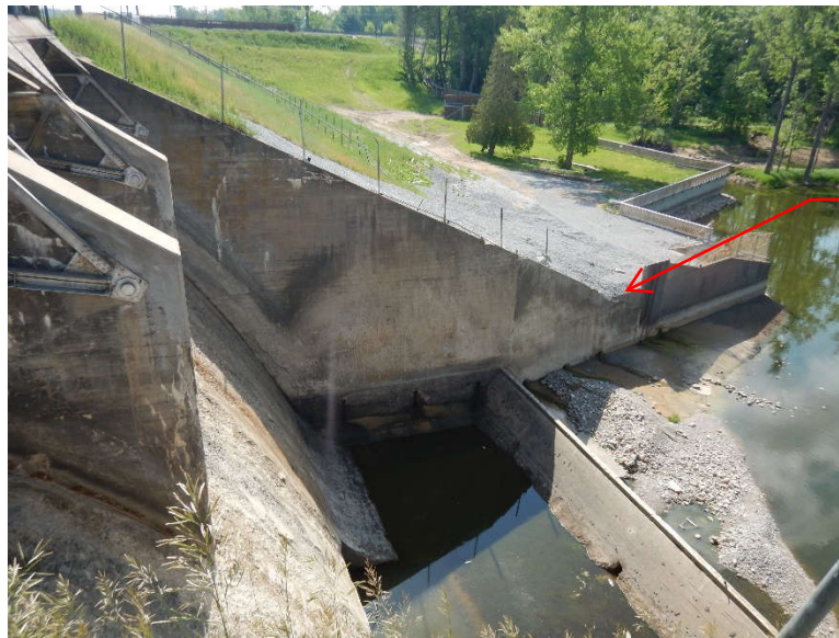
Photo 30: Left side (east) retaining wall exhibiting cracking with efflorescence, several large spalls near the bottom and a steel plate reinforcing an area under construction.
