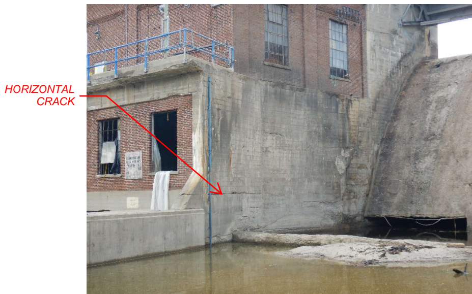
Photo 17: Powerhouse foundation with large crack and missing windows.
