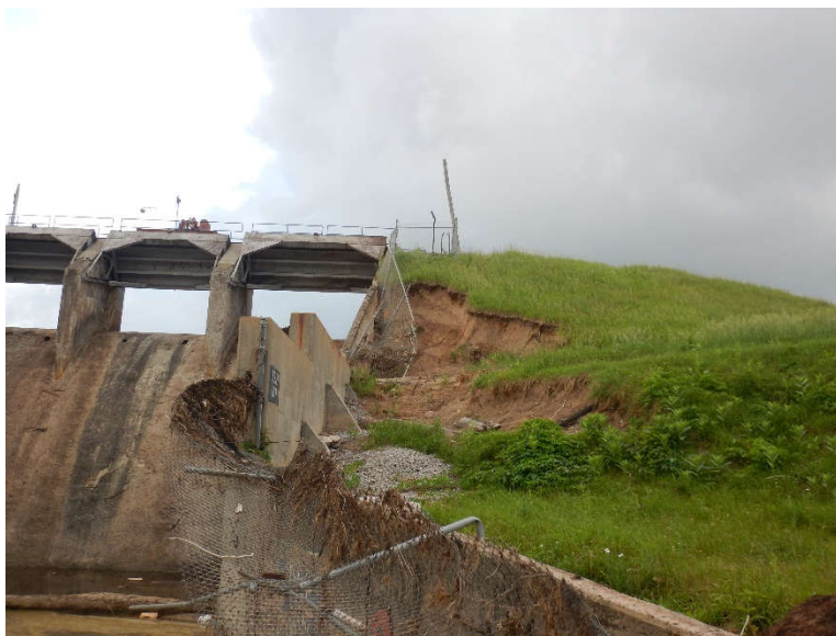
Photo 13: Erosion behind left side (east) retaining wall at downstream end.
