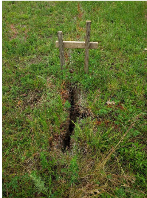
Photo 46: Boyce Hydro installed crack gauges to monitor the tension cracks.
