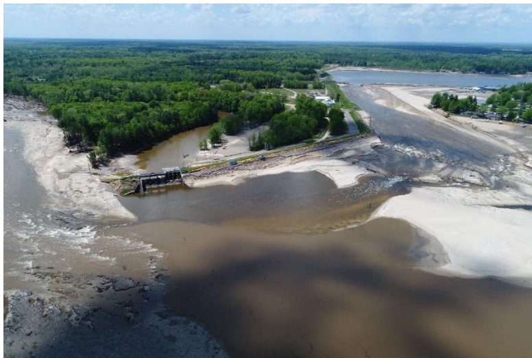
Photo 20: Upstream slope of the Right Embankment – Tittabawassee (drone photo provided by EGLE).
