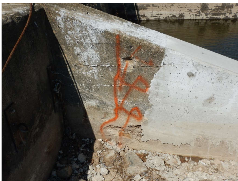
Photo 35: Upstream left side (east) retaining wall with delamination near recent patch (2'x4')
