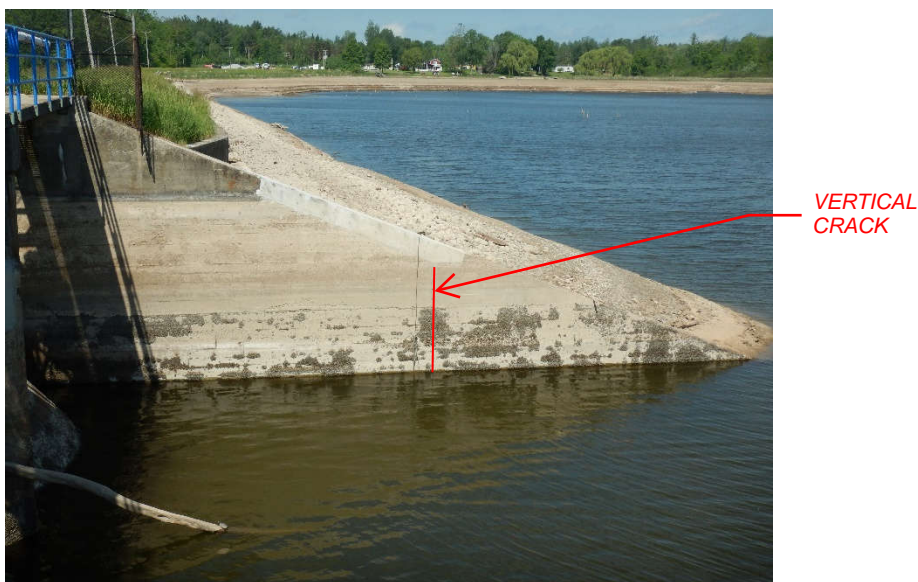
Photo 34: Upstream right side (west) retaining wall with a crack just right of the vertical line (cable hanging over edge).
