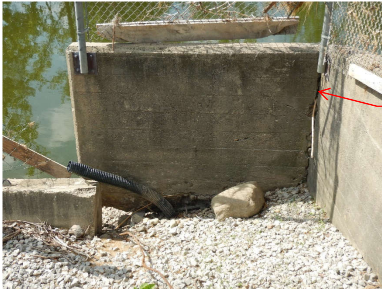
Photo 39: Left (east) side cutoff wall with fully cracked connection to retaining wall and large spall with exposed reinforcing steel.
