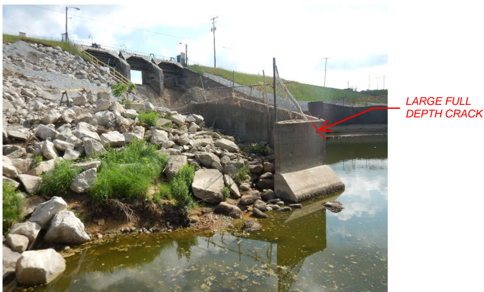
Photo 40: Right (west) side cutoff wall with large crack near top at connection with retaining wall. Also note the lack of backfill
