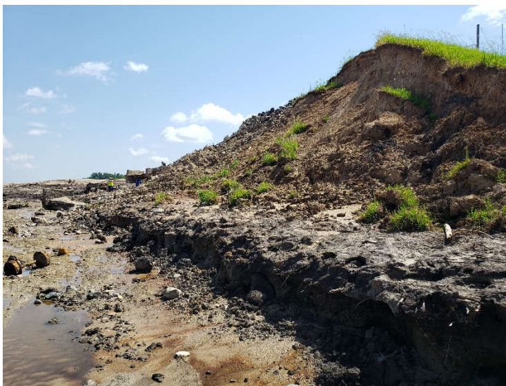
Photo 2: Left section of embankment that has eroded and requires stabilization.
