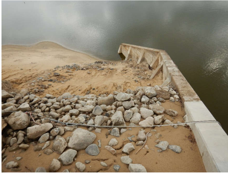
Photo 11: Erosion behind right side (west) retaining wall at upstream end.
