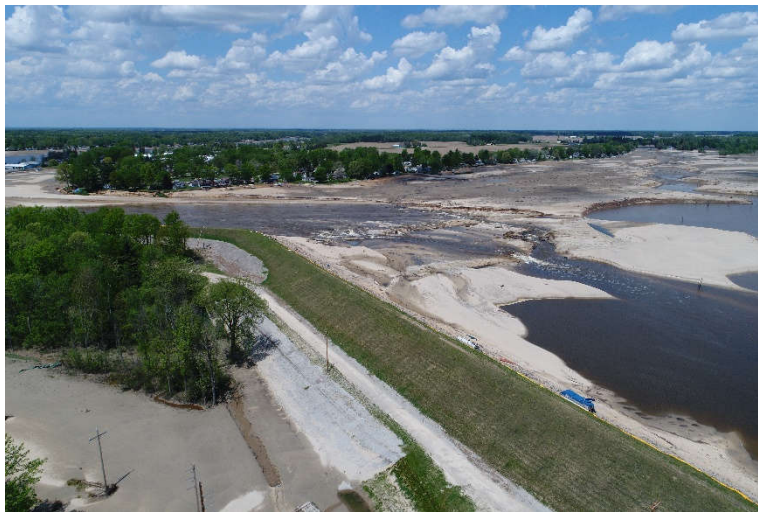
Photo 22: Downstream slope of Right Embankment – Tittabawassee (drone photo provided by EGLE).
