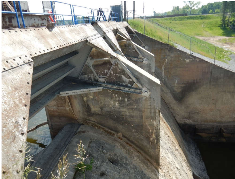
Photo 28: Tobacco spillway pier with recent patch and still showing cracking with efflorescence.
