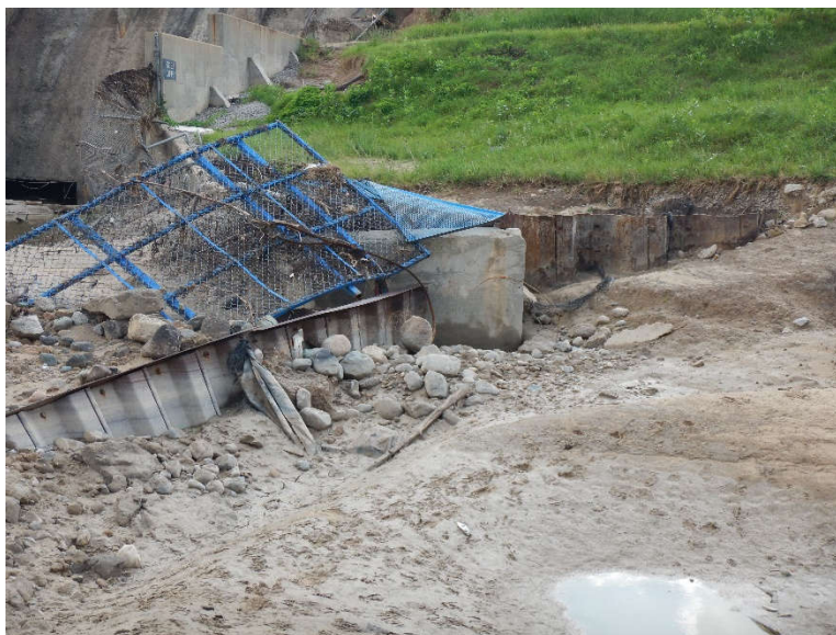
Photo 15: Left side (east) cutoff buried under debris. Note failure of supporting sheet pile wall in the foreground.
