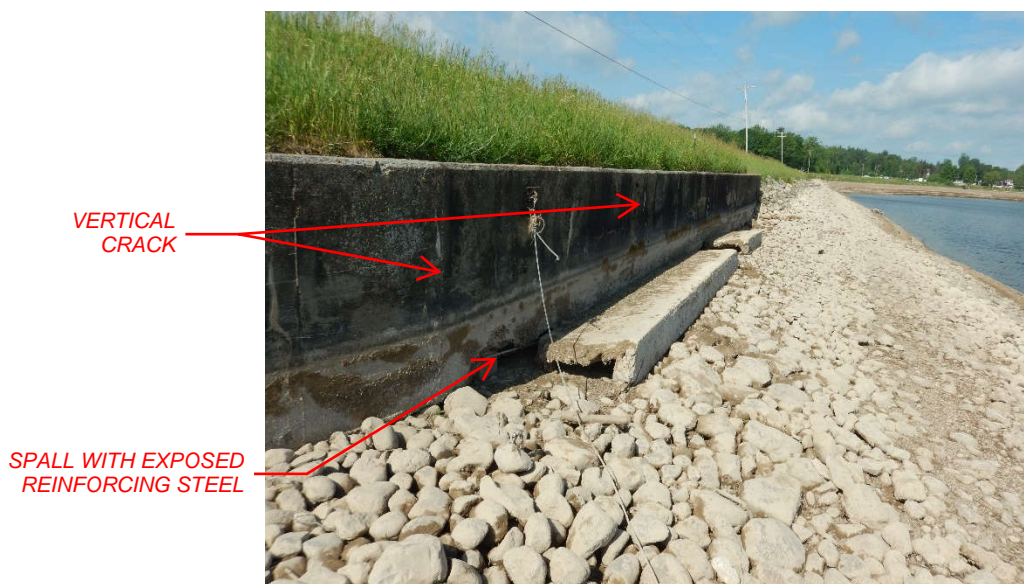
Photo 36: Right side (west) wingwall (bulkhead) with vertical cracks and spalls exposing the sheet piling and reinforcing steel.
