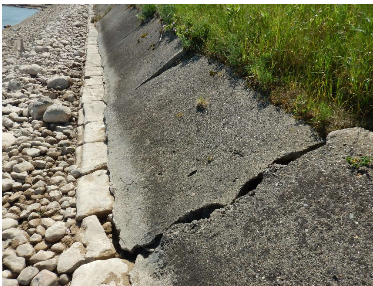
Photo 37: Concrete slope protection panel approximately 40' east of the wingwall (bulkhead) with undermining and settlement present.
