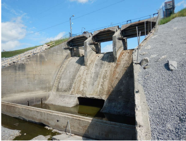
Photo 27: Tobacco spillway with widespread spalling and likely delamination
