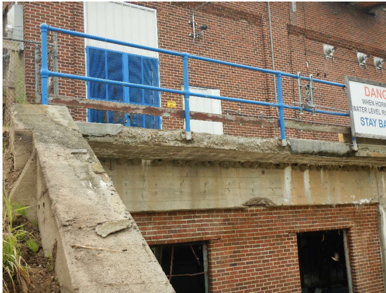
Photo 18: Powerhouse back porch with significant spalling on edge of slab.
