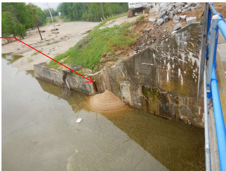
Photo 8: Right side (west) downstream retaining wall showing cracks, efflorescence and leaking backfill. Note the horizontal extension is separated from the main wall at the toe of the slope and rotated towards the stream.
