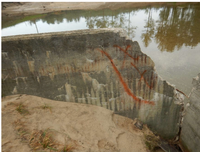
Photo 9: Portion of right side (west) retaining wall missing with areas of delamination, cracking with efflorescence and erosion.
