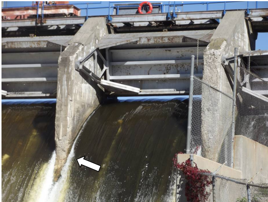
Photograph 28 – Center gate of Tittabawassee spillway. Note the moderate spalling of pier nose.
