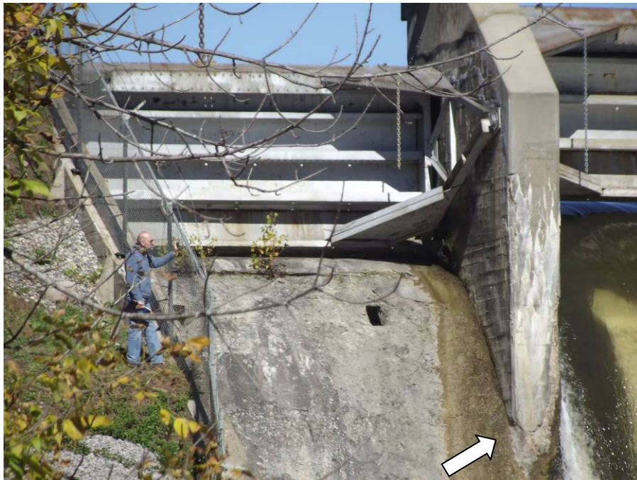
Photograph 12 – Right gate of Tobacco spillway. Note the moderate spalling of pier nose and spillway face.
