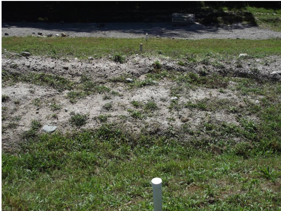
Photograph 8 – Piezometers at right Tobacco embankment.
