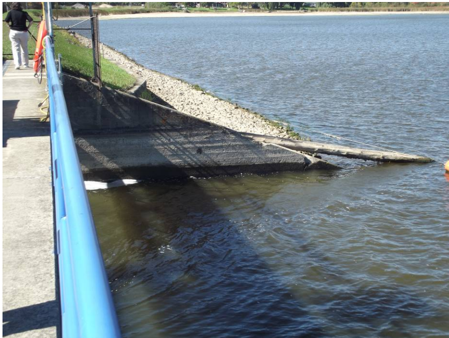
Photograph 14 – Right upstream abutment wall of Tobacco spillway. Note the moderate spalling at the top of wall.
