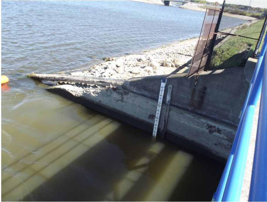
Photograph 13 – Left upstream abutment wall of Tobacco spillway. Note the significant spalling and exposed reinforcing steel at top of wall.
