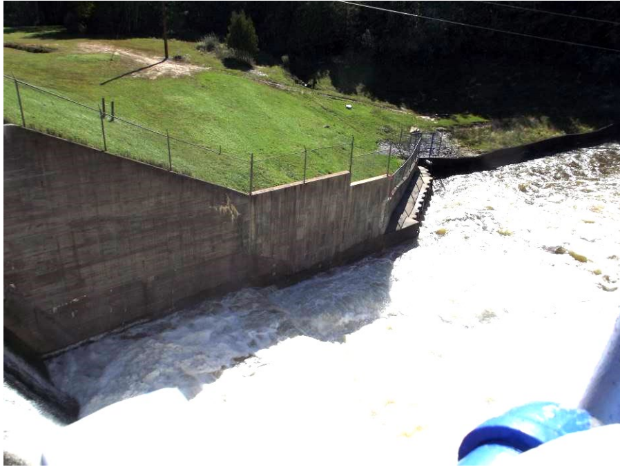
Photograph 33 – Downstream left abutment wall of Tittabawassee spillway.
