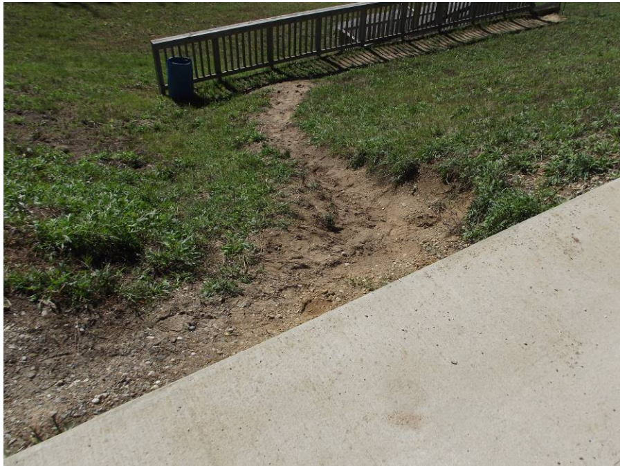
Photograph 4 – Foot traffic erosion at left Tobacco embankment.
