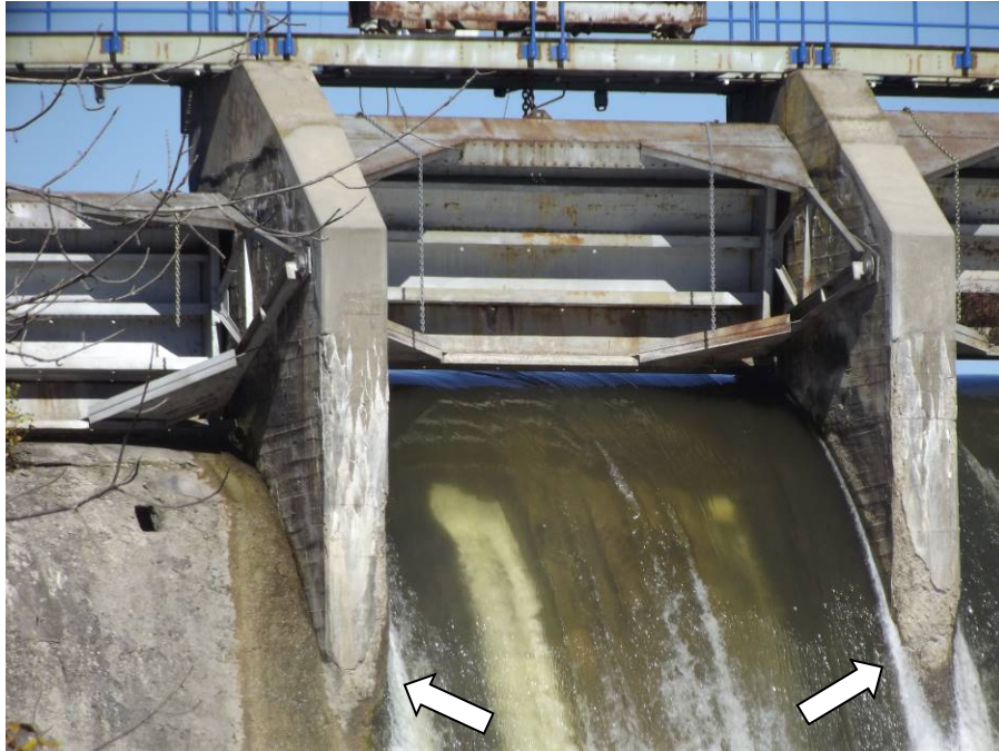
Photograph 11 – Center gate of Tobacco spillway. Note the moderate spalling of pier noses.
