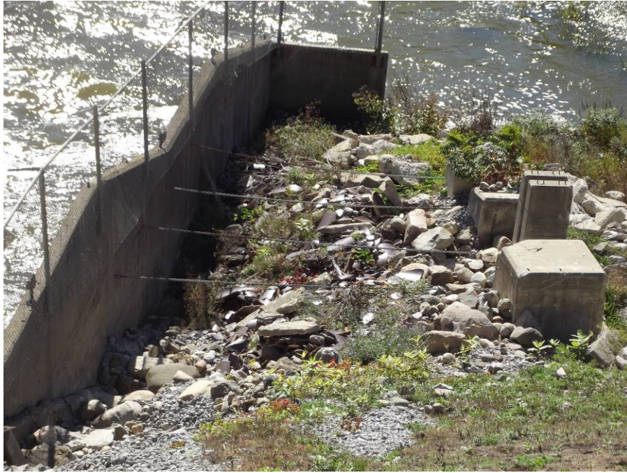
Photograph 19 – Erosion behind right abutment wall. Note the dead men and tie-backs and rotation of lower wall.
