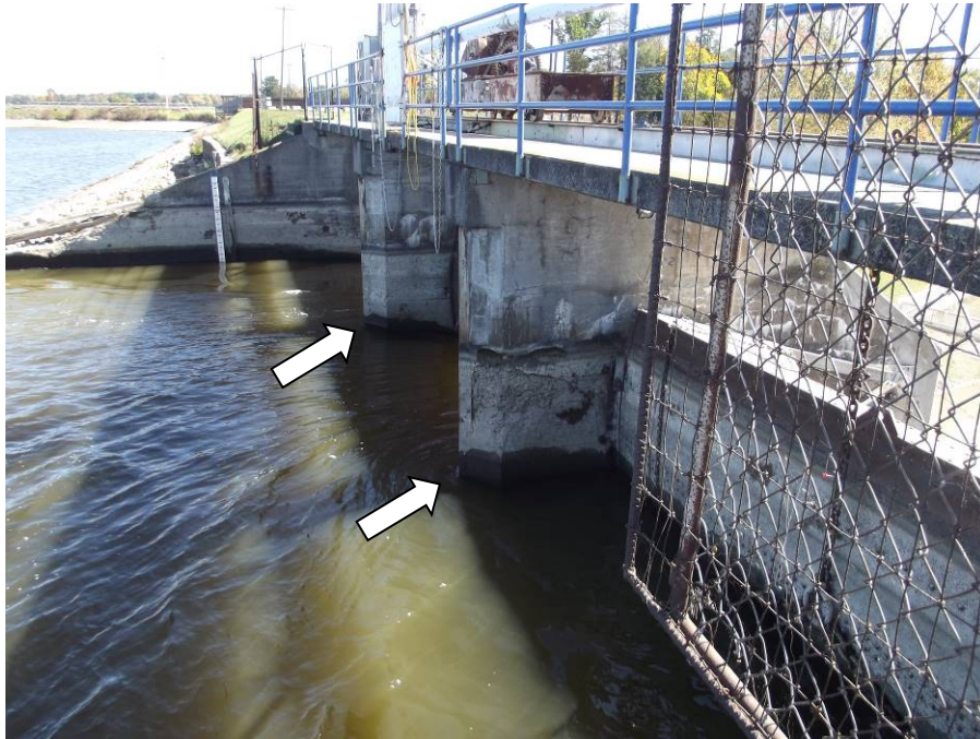
Photograph 15 – Upstream face of Tobacco spillway. Note the moderate spalling of pier noses.
