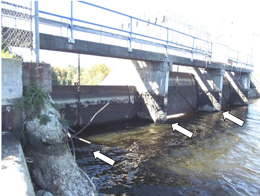
Photograph 35 – Upstream face of Tittabawassee spillway. Note the significant spalling and exposed reinforcing steel throughout.
