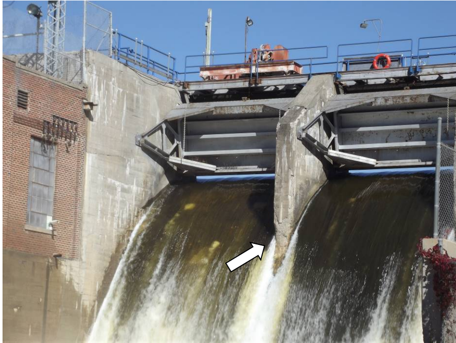
Photograph 27 – Right gate of Tittabawassee spillway. Note the moderate spalling of pier nose.
