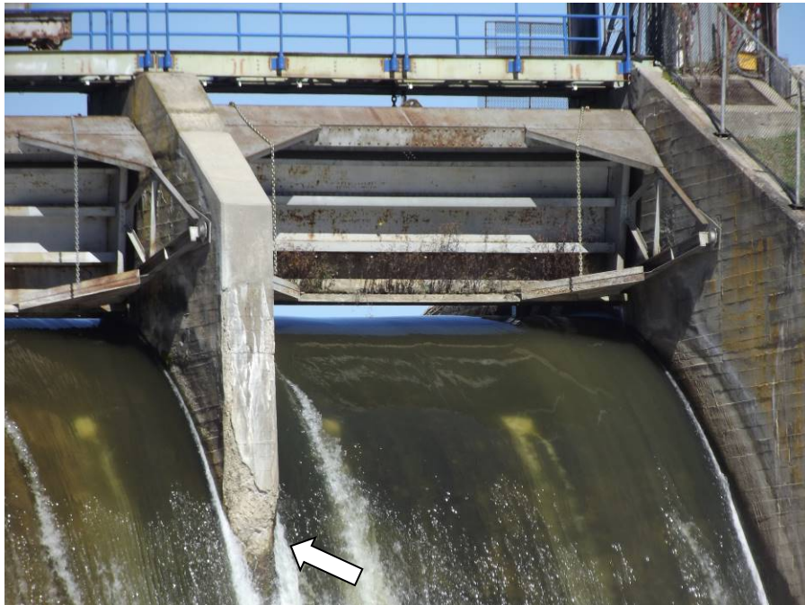
Photograph 10 – Left gate of Tobacco spillway. Note the moderate appalling of pier nose.
