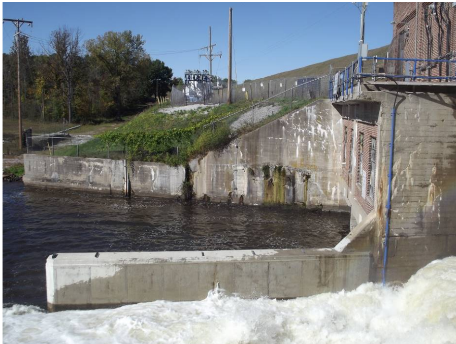
Photograph 32 – Downstream right abutment wall of Tittabawassee spillway. Note the significant spalling, cracking and efflorescence throughout.
