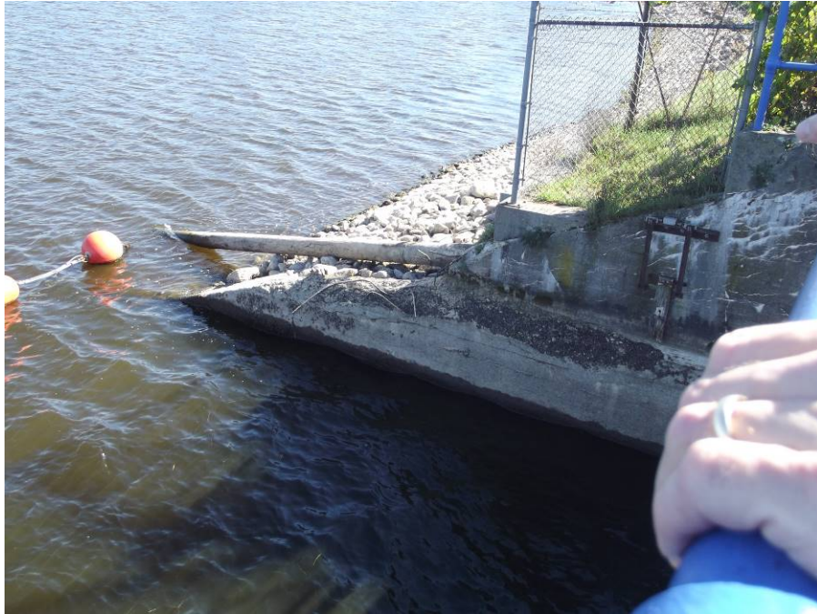
Photograph 31 – Upstream left abutment wall of Tittabawassee spillway. Note the significant spalling and exposed reinforcing steel at top of wall.
