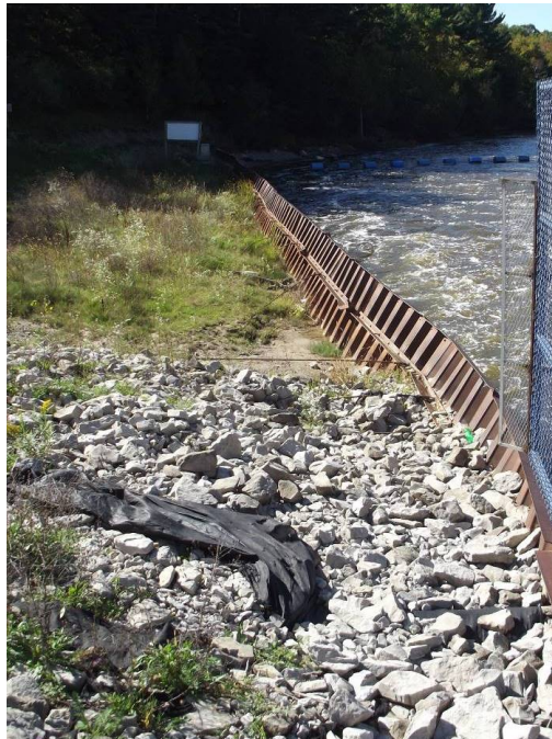
Photograph 34 – Failing retaining wall downstream of left abutment.
