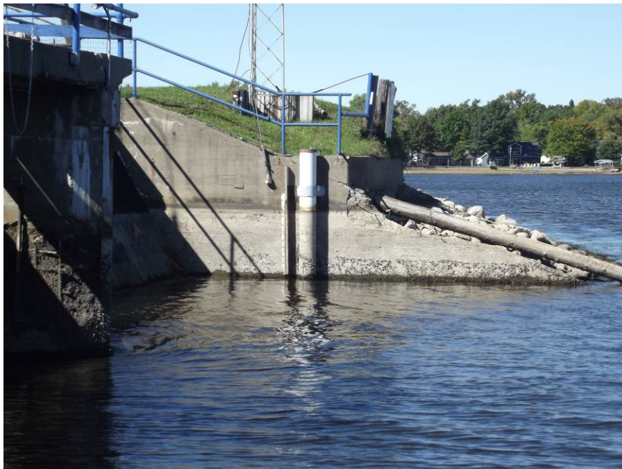
Photograph 30 – Upstream right abutment wall of Tittabawassee spillway. Note the significant spalling and exposed reinforcing steel at top of wall.
