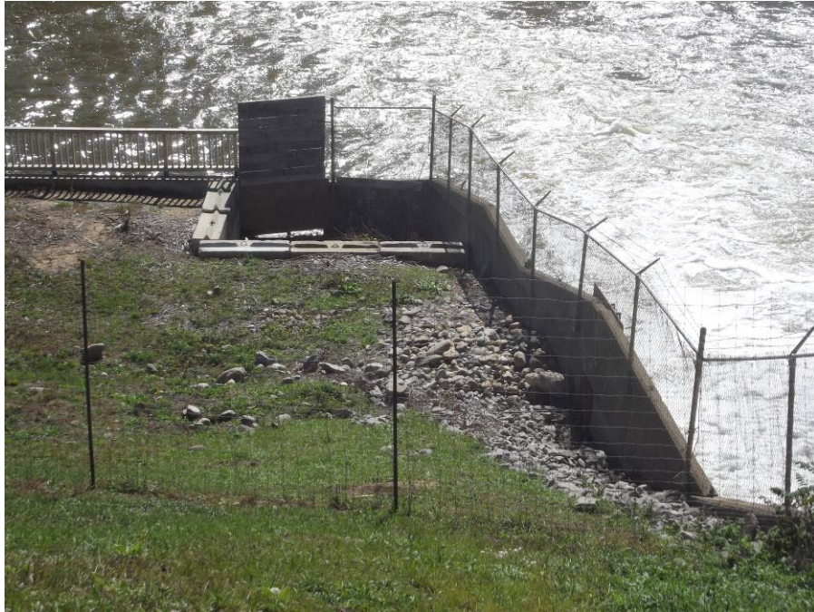
Photograph 17 – Erosion behind left abutment wall.
