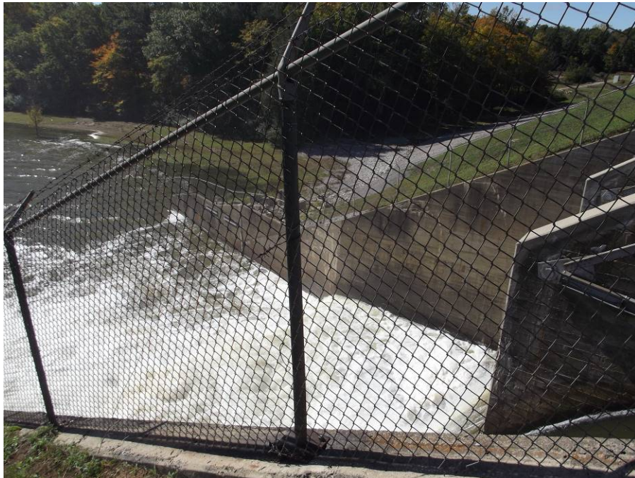
Photograph 18 – Downstream right abutment wall of Tobacco spillway.
