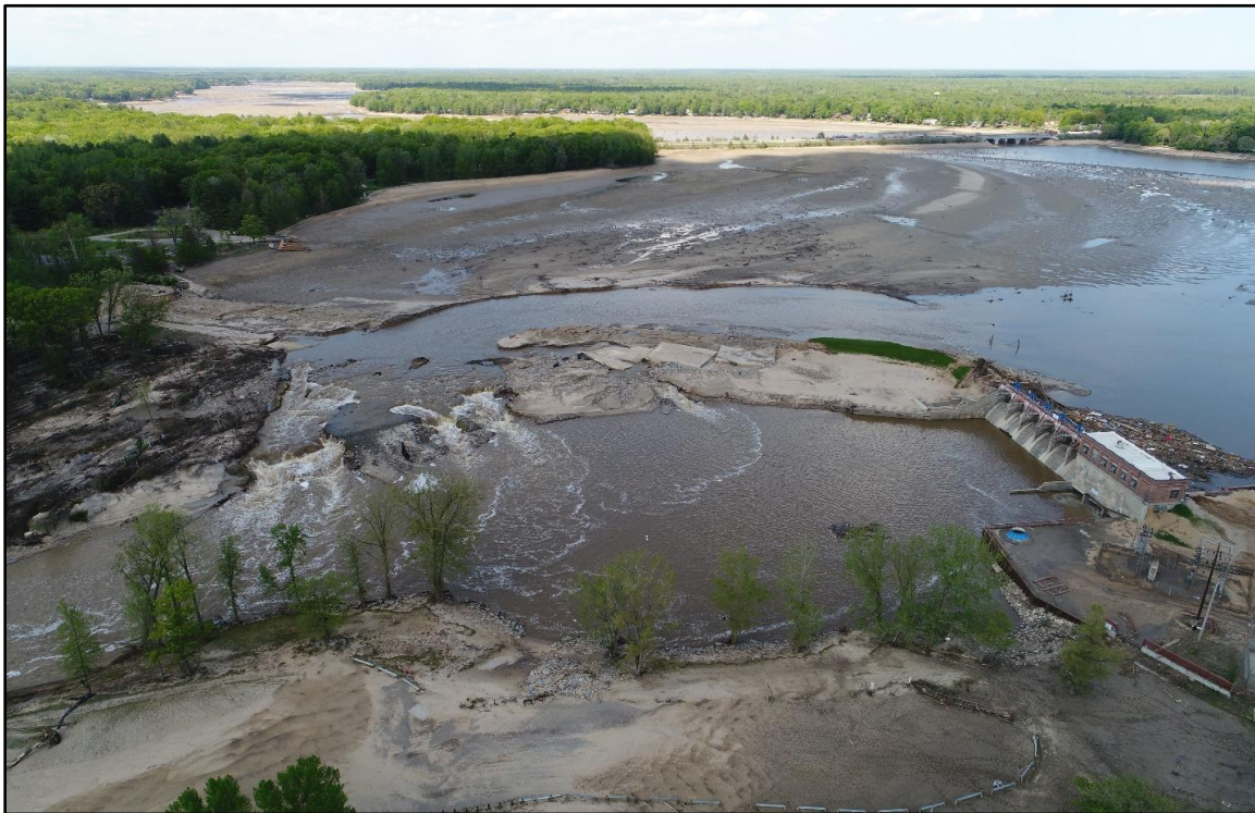
Figure 2: Aerial photograph of the failed Sanford Dam, looking north, taken on May 26, 2020. On Tuesday, May 19, 2020, an estimated 200-year weather event caused local rivers to swell, especially in Arenac, Bay, Gladwin, Iosco, Midland, and Saginaw Counties. Flood waters caused additional stress on local dams and contributed to the failure of the Edenville and Sanford Dams and caused damage to the Chappel, Beaverton, Secord, Smallwood, and Forest Lake Dams. Failure of the two dams released a torrent of water, devastating the downstream communities of Edenville, Sanford, Midland, and Saginaw.
