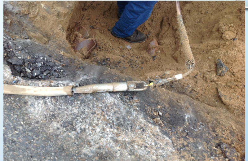
Copper Line Connected to Pulling Harness
