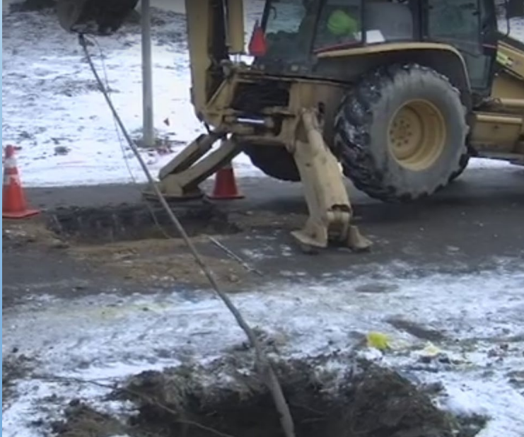
Backhoe – Pulling Line Through
