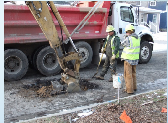
Excavation at Main
