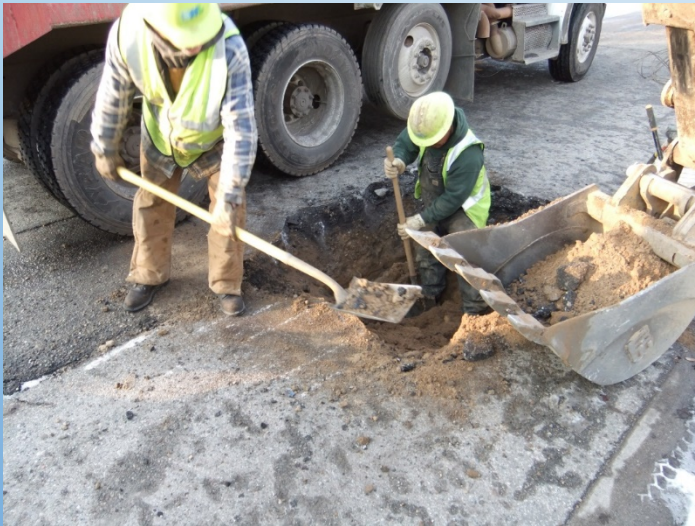
Excavation at Curb Stop
