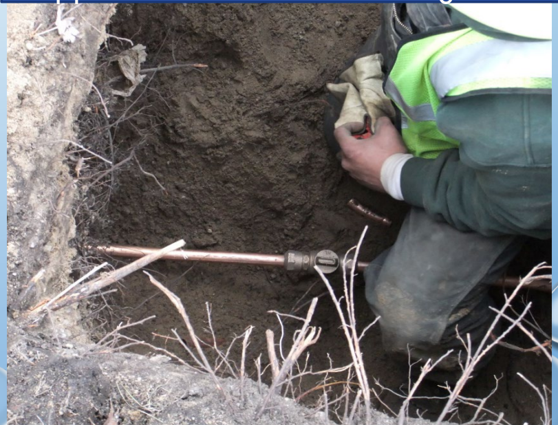
Finishing up Attaching Copper Line
