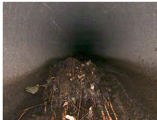
Figure 1: Roots and Deposits in Pipe
