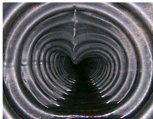
Figure 4: Deformed Culvert
