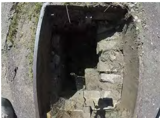
Figure 2: Deteriorated Stormwater Inlet
