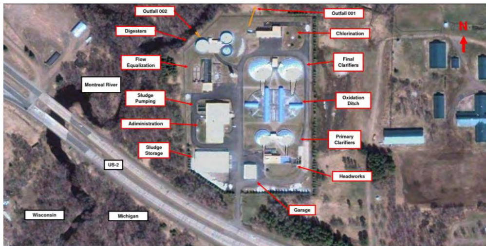
Figure 1 GIWA Treatment Plant
