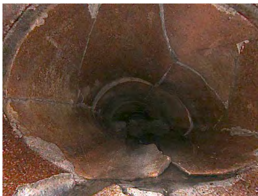
Figure 3: Collapsing Clay Pipe
