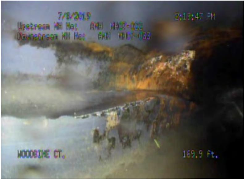
Figure 7. Defect Example: Deformed Flexible Inverse Curvature.
