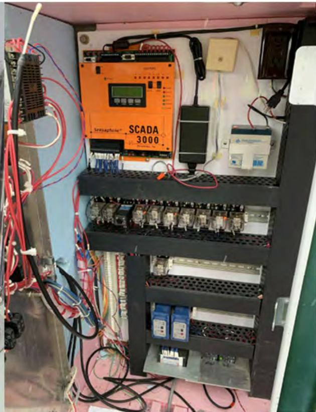
Figure 5: SCADA Control Board at the Ashford Pump Station
