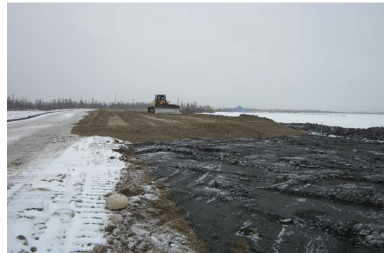
Sand and gravel over thickened tailings
