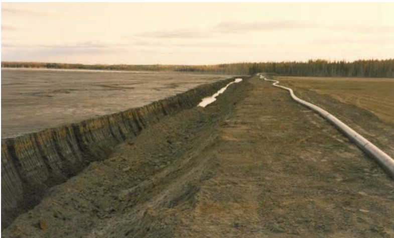
After upstream dyke raise is complete
