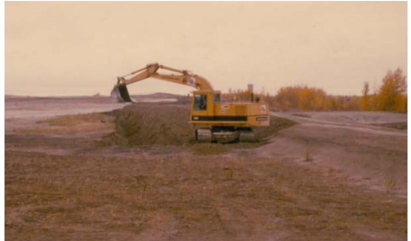
Tailings excavation during upstream dyke raise
