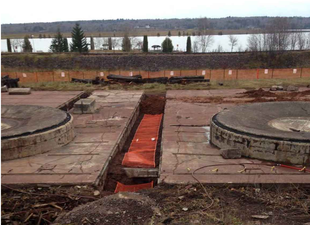
Photo 4: Demarcation layer in the deep trench
