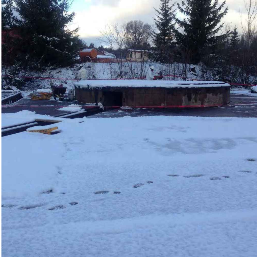
Photo 38: Preparing to remove pitch mastic from floatation tank foundation after snow
