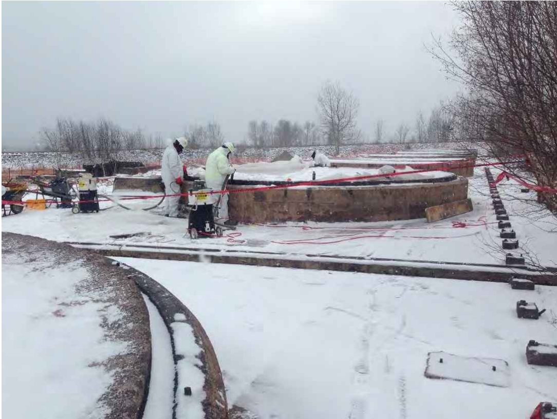
Photo 40: Equipment setup for pitch mastic removal.
