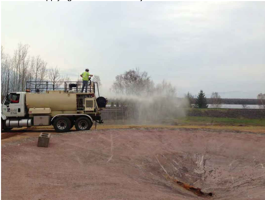
Photo 63: Applying tackifier to east adjacent excavated area
