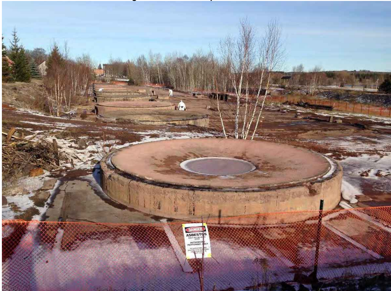
Photo 24: Cleaning the Calumet Stamp Mill trenches and foundation
