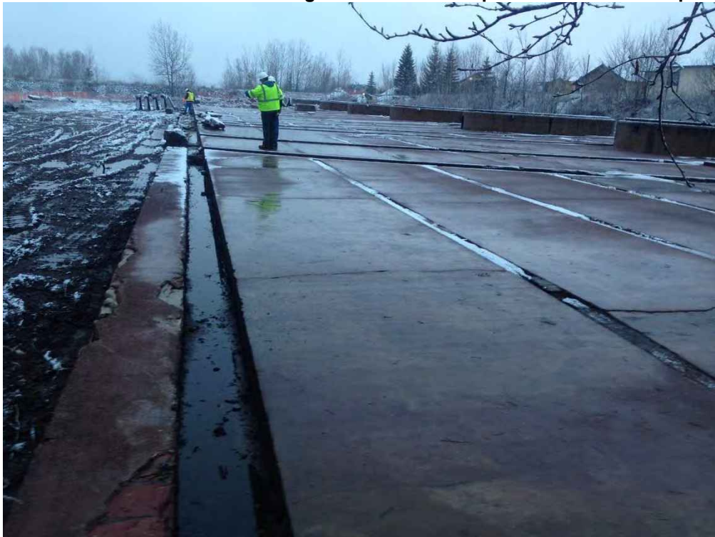
Photo 6: Excavation of eastern edge of Calumet Stamp Mill foundation complete
