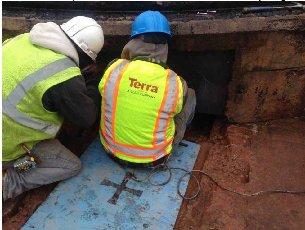
Photo 5: Steel plate installation in floatation tank foundation openings.
