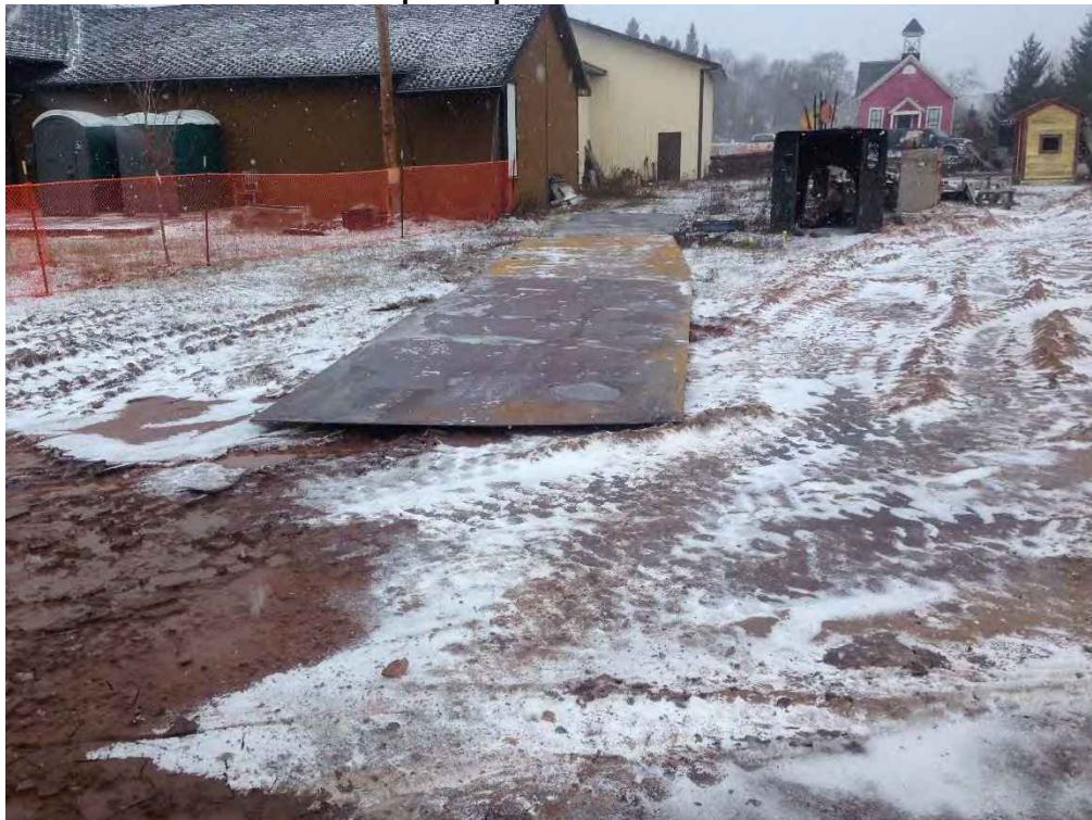
Photo 8: 8x20' Steel plates placed over tunnel area for HCHMS.
