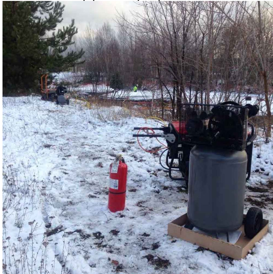
Photo 40: Equipment setup for pitch mastic removal.
