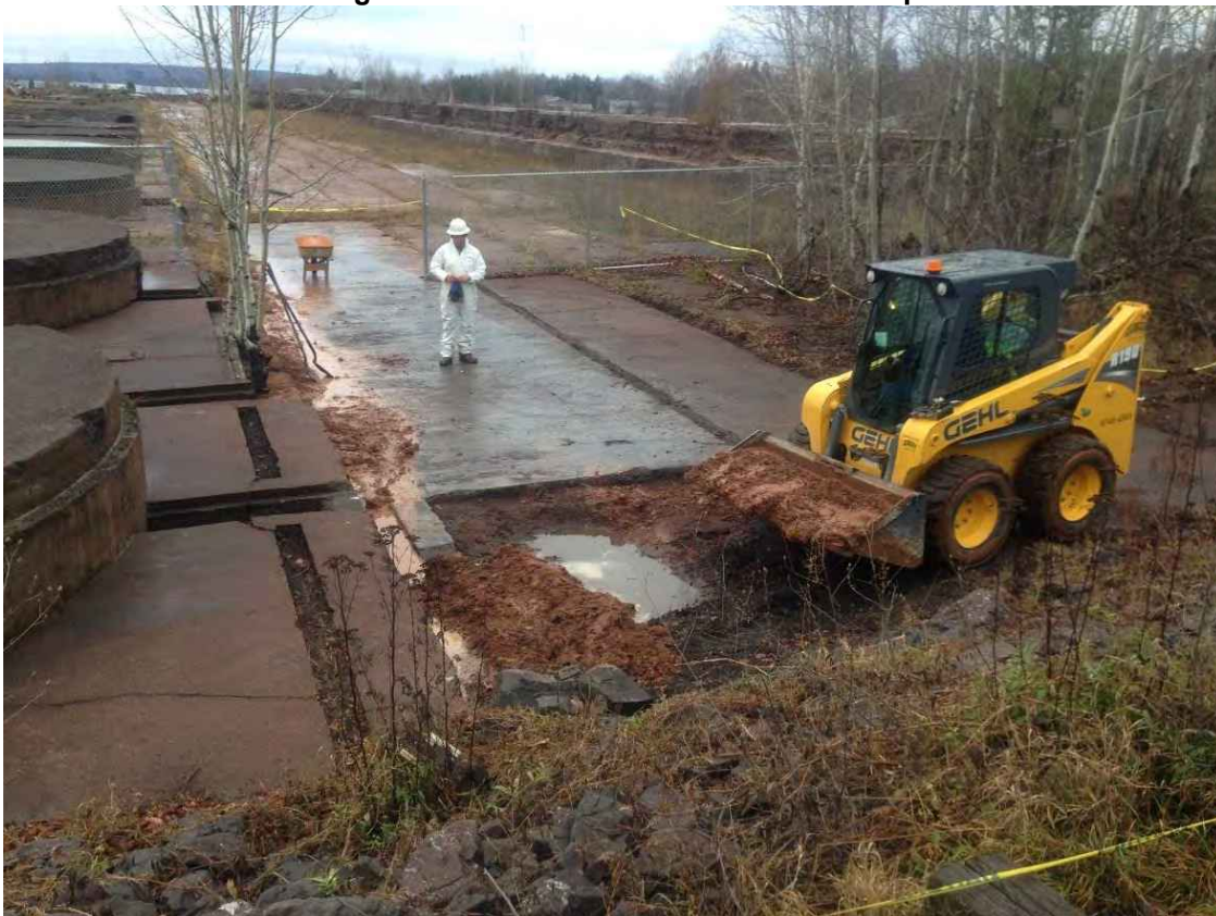
Photo 28: Backfilling holes and trenches on the Hecla Stamp Mill foundation.
