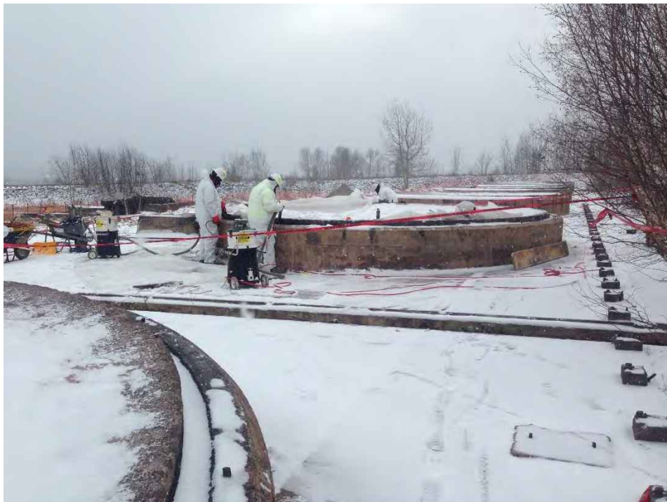
Photo 2: Pitch mastic removal in the snow
