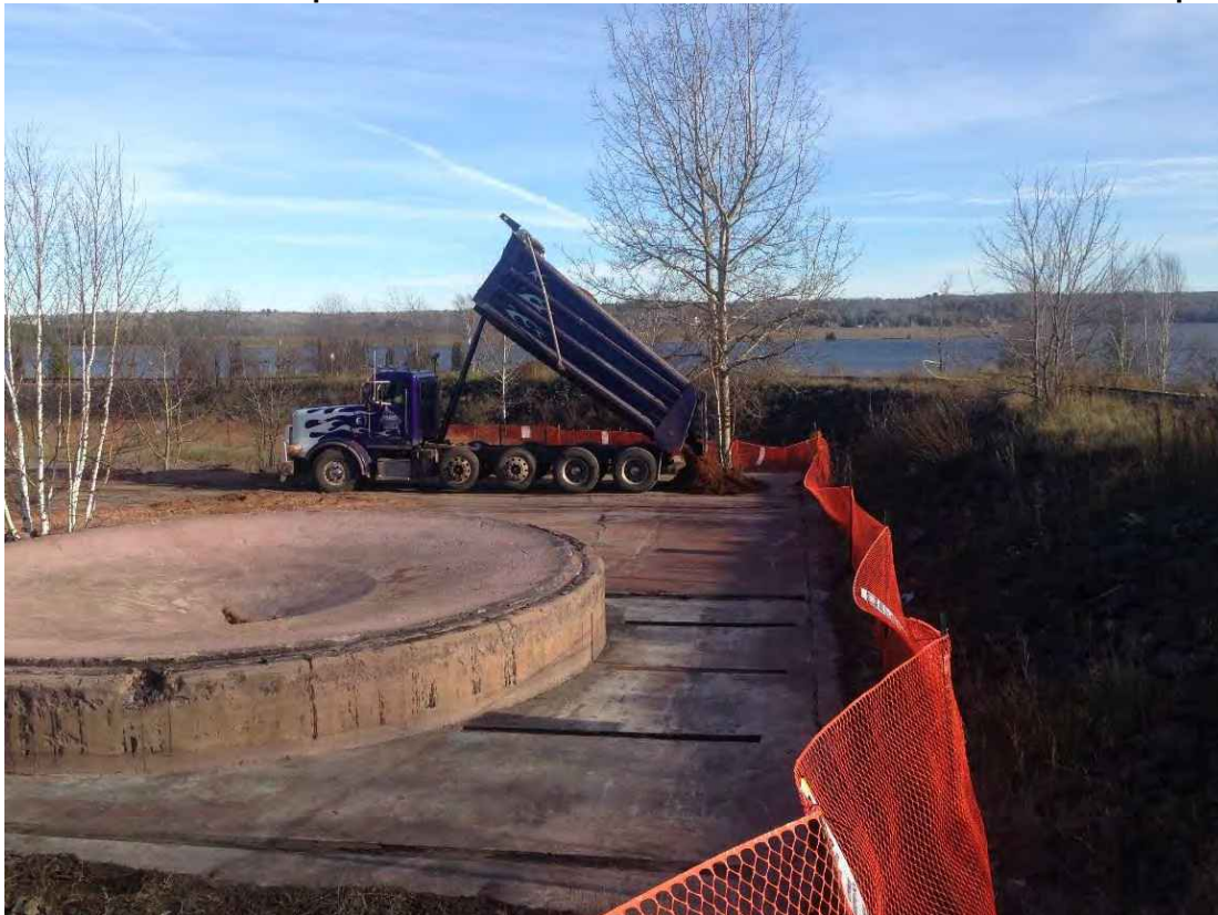
Photo 12: Place clean topsoil backfill on the southeastern corner of the Calumet Stamp Mill.
