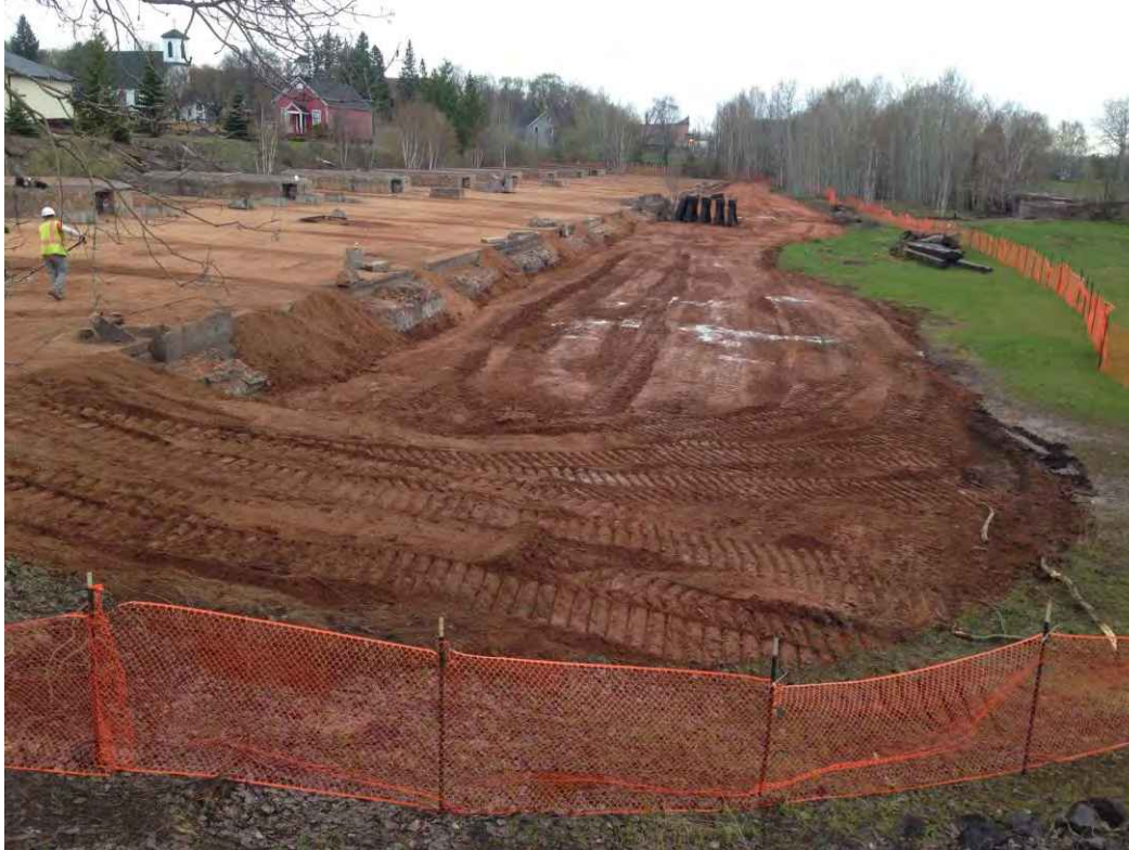
Photo 58: East adjoining excavated area backfilled with 6-inches of “top soil”
