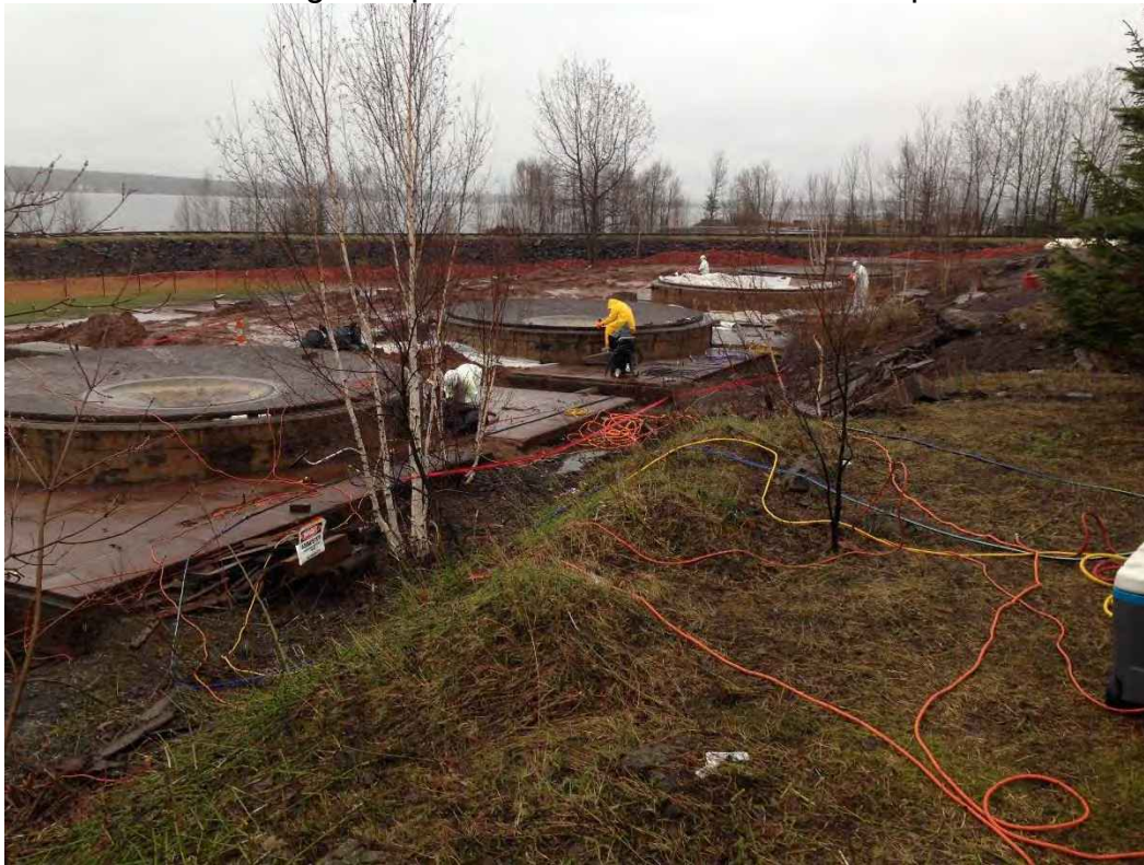
Photo 52: Final stages of pitch mastic removal and cleanup
