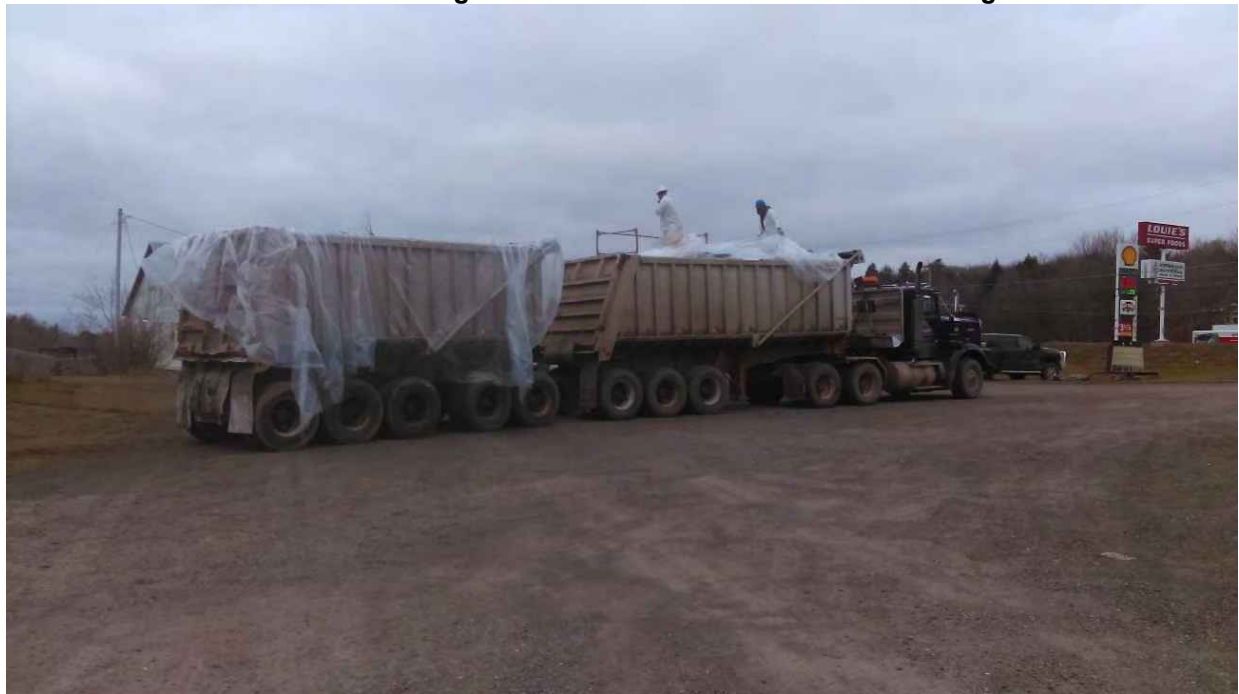
Photo 16: Sealing the material within truck beds after filling
