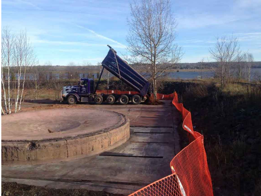
Photo 4: Dust control during Calumet Stamp Mill cleaning
