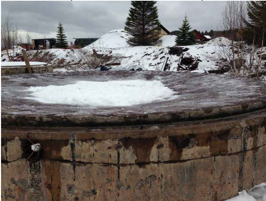
Photo 53: Final inspection of floatation tank foundation pitch mastic removal
