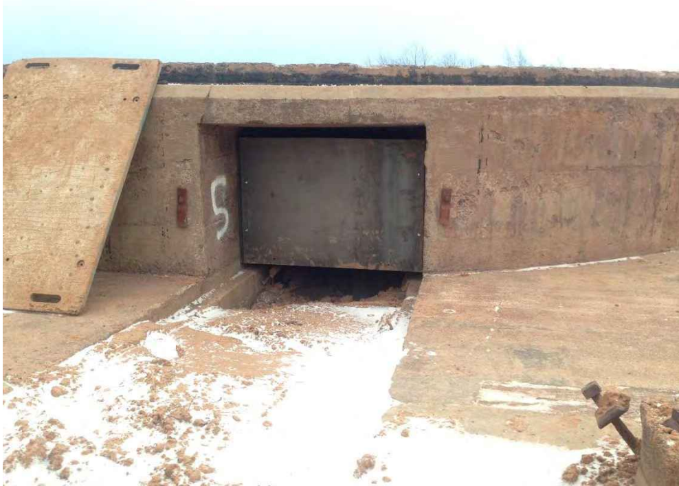
Photo 6: Typical steel plate installation in the floatation tank foundation openings
