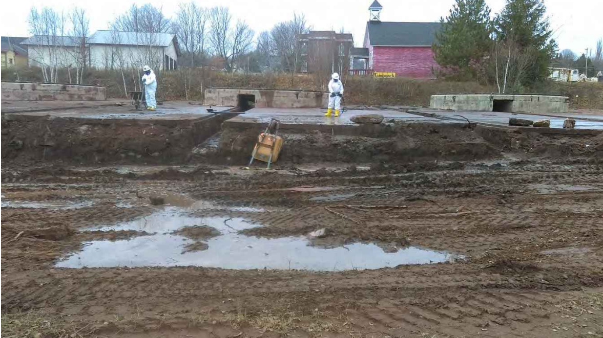
Photo 5: Washing the northern portion of the Calumet Stamp Mill foundation.
