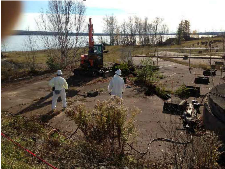
Photo 2: Removing trees from the Hecla Mill foundation
