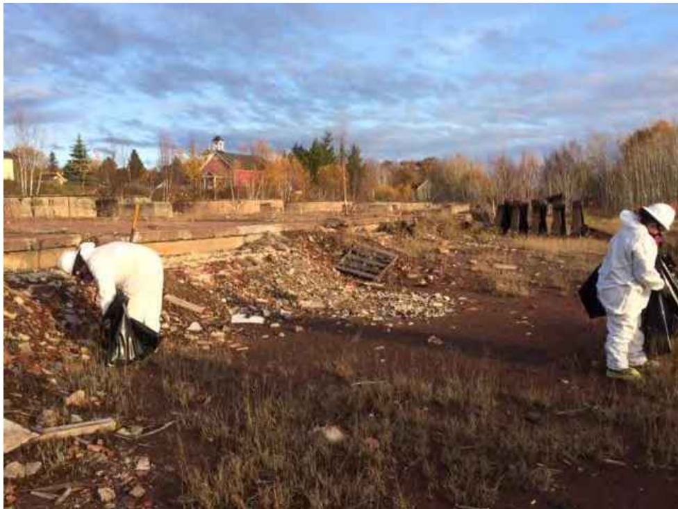
Photo 4: Surficial Asbestos Removal
