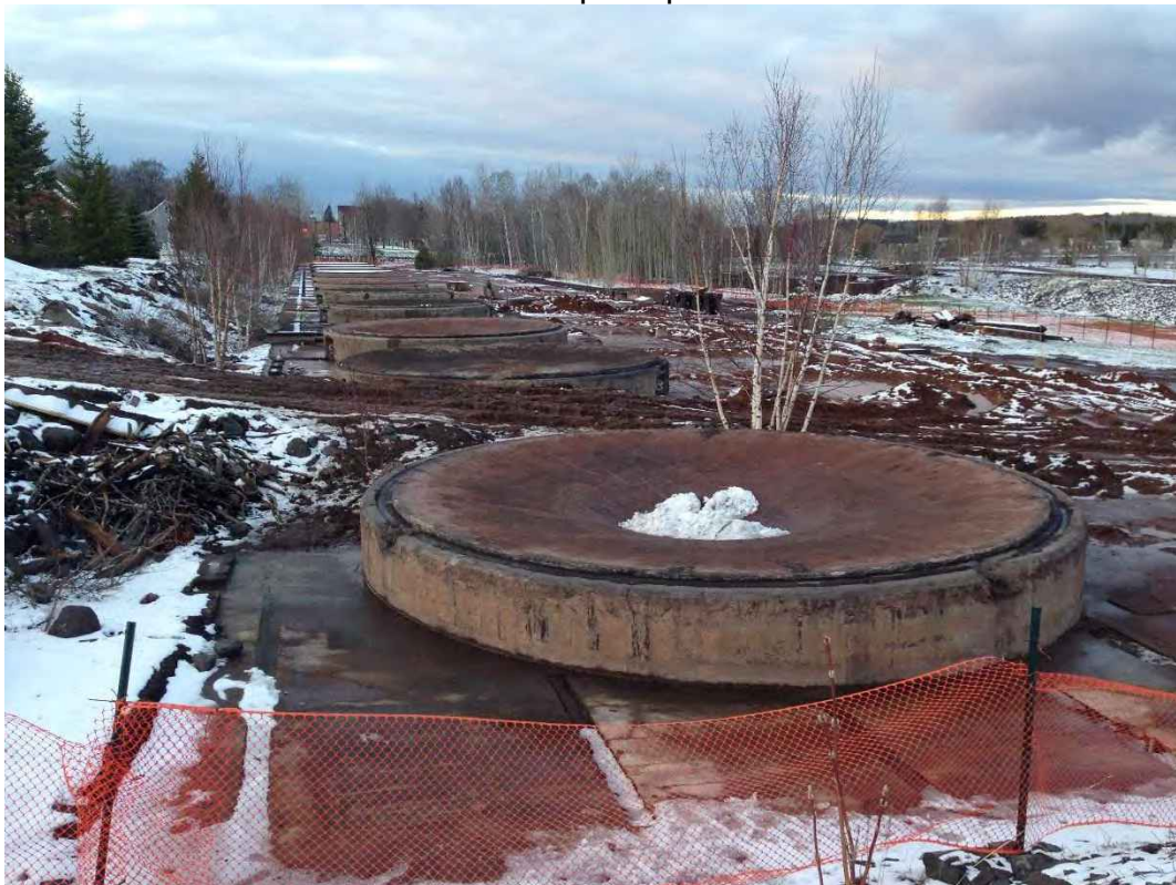
Photo 55: Pitch mastic removal complete per START contractor
