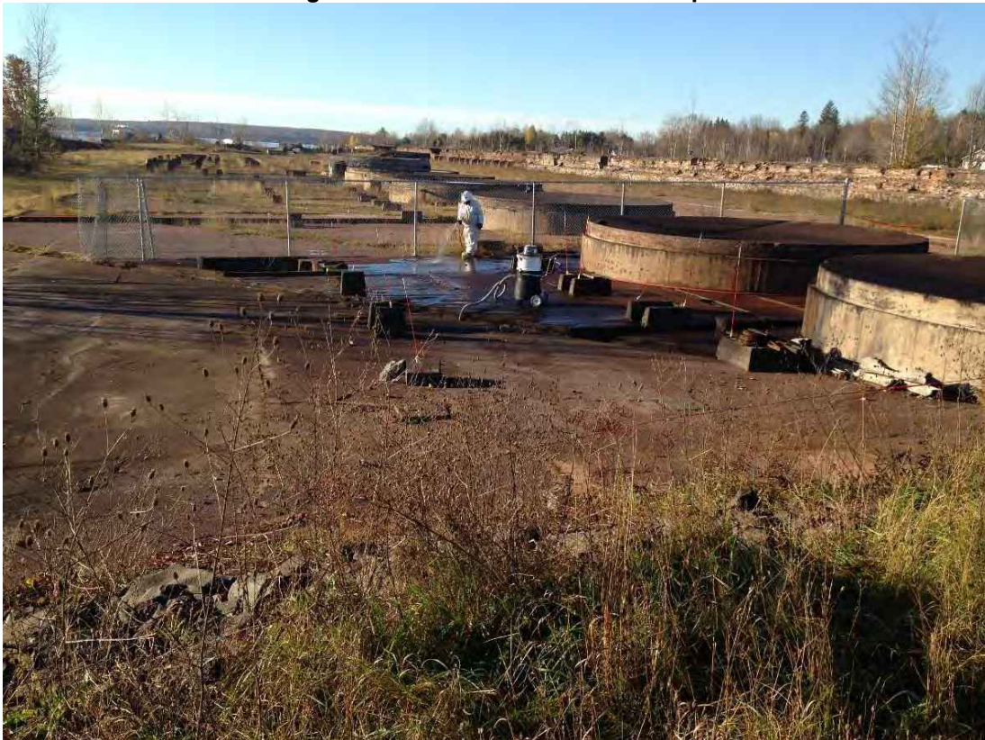
Photo 10: Cleaning the North end of the Hecla Stamp Mill Foundation
