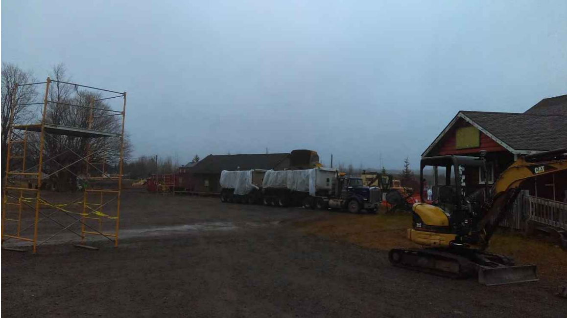
Photo 1: Loading plastic sheeting lined trucks with possible asbestos containing material
