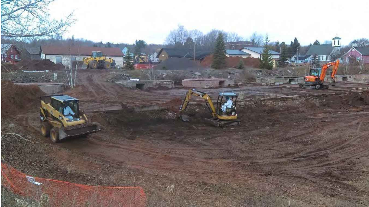
Photo 18: Excavation of the eastern edge of the Calumet Stamp Mill nearly complete
