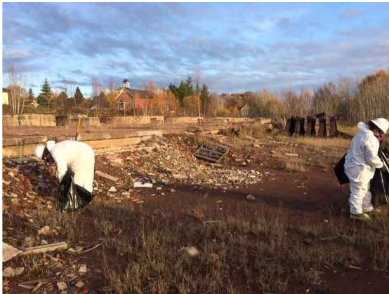
Photo 4: Surficial Asbestos Removal
