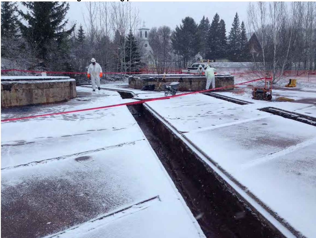
Photo 36: Begin removing pitch mastic from flotation tank foundations.
