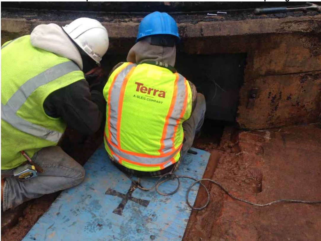
Photo 42: Steel plate installation in floatation tank foundation openings.
