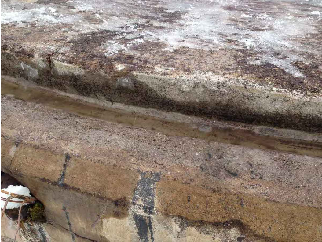
Photo 54: Final inspection of floatation tank foundation pitch mastic removal
