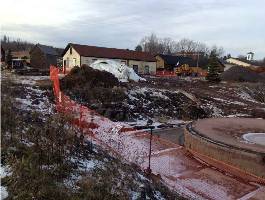
Photo 28: Backfilling holes and trenches on the Hecla Stamp Mill foundation.
