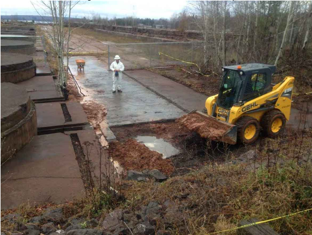
Photo 1: Backfilling holes and trenches on the Hecla Stamp Mill foundation
