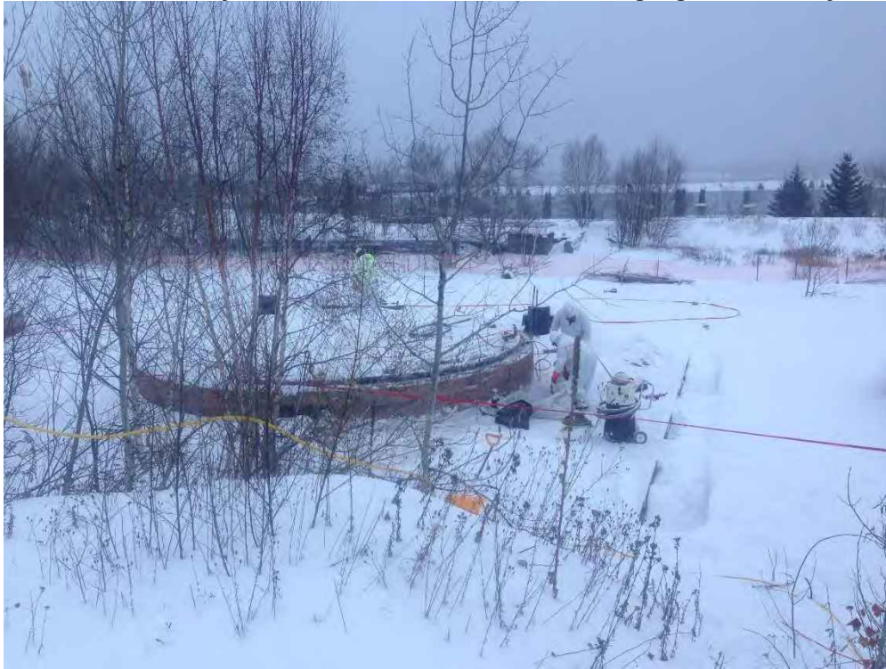
Photo 8: 8x20' Steel plates placed over tunnel area for HCHMS.
