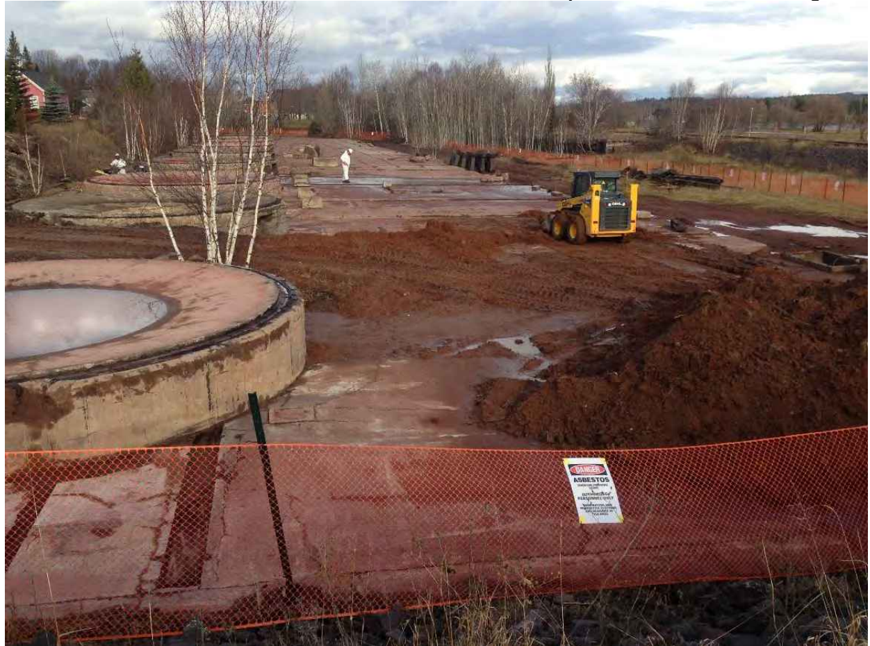
Photo 30: Trenches and surface clean on the Calumet Stamp Mill foundation: Backfilling.
