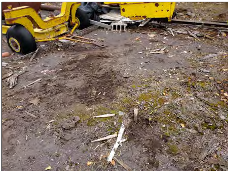
Photo 7: View of the ground surface after being scraped to remove scattered TSI at Julio Contracting/Formers Standard Oil Co.
