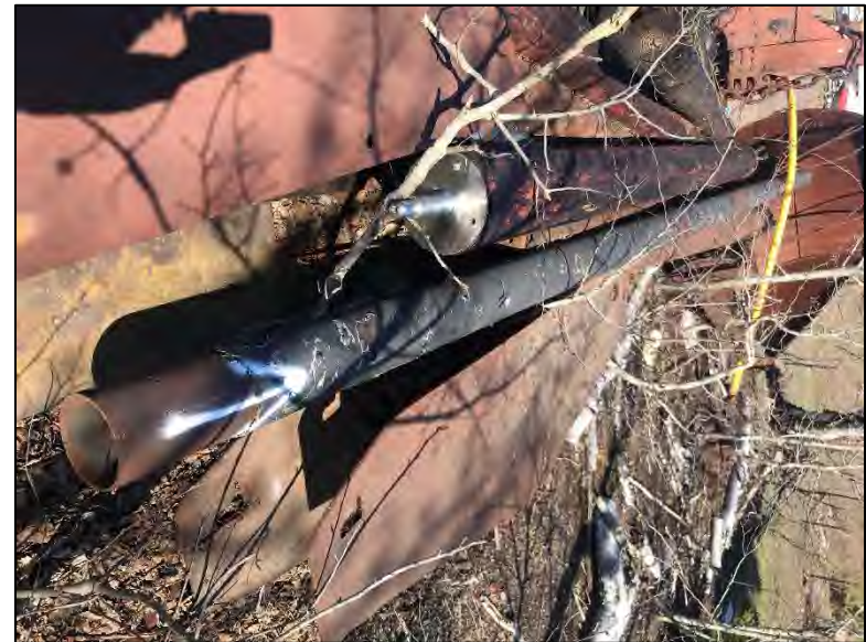
Photo 12: View of a pipe wrapped in ACM, identified with marking paint, which was cut up and removed from Julio Scrap Yard & Tower.
