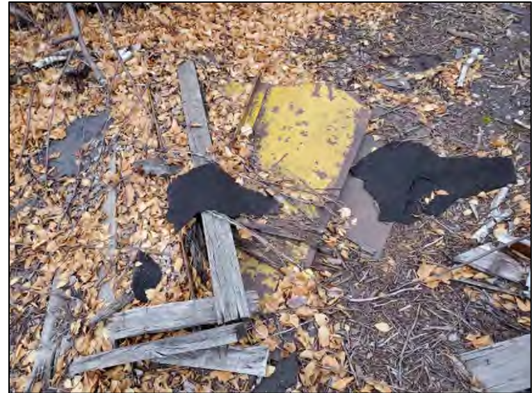
Photo 2: View of scattered suspect ACM roofing materials which have been removed at Julio Contracting/Former Standard Oil Co.
