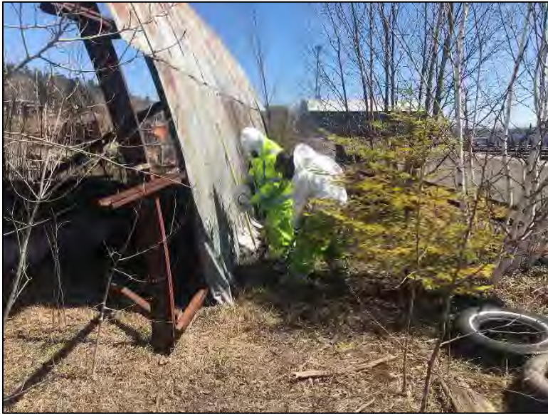
Photo 9: View looking east of non-friable ACM roof coating being picked up along a structure near the MDNR Trail at Julio Contracting/Former Standard Oil Co.
