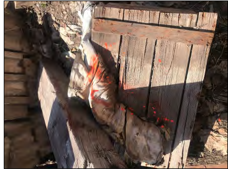
Photo 10: View of suspect ACM, marked with marking paint, removed near the office at Julio Contracting/Former Standard Oil Co.
