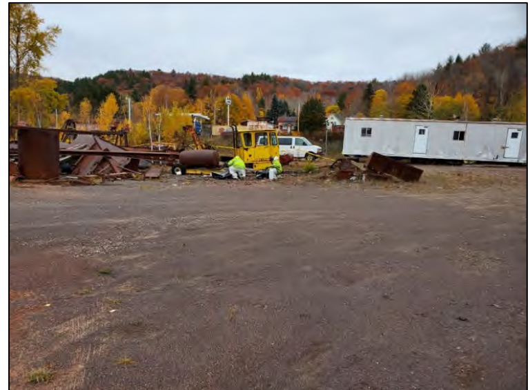
Photo 4: View looking north of scattered TSI being wetted and scraped from the ground surface using hand tools at Julio Contracting/Former Standard Oil Co.
