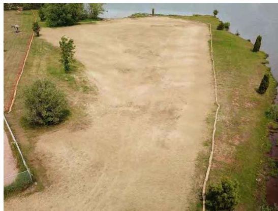
Seeded and Mulched Ground Surface
