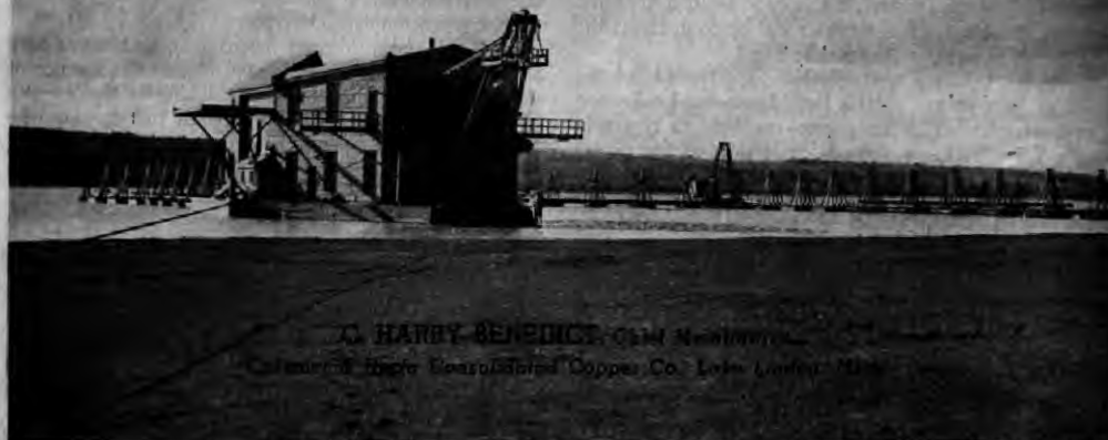
NEW SUCTION DREDGE at work on Quincy's bank of amygdaloid sands in Torch Lake. The suction pipe, which is carried on the pontoons, delivers to the screen at the storage pool at the shore plant
