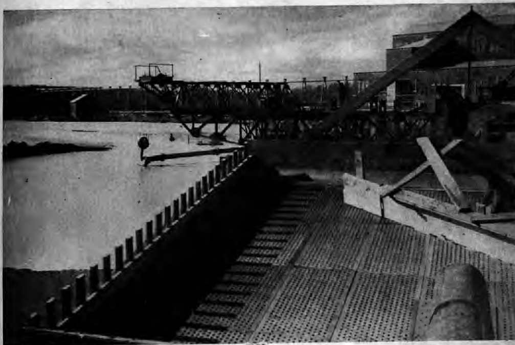
AT THE STORAGE POOL the sands delivered from the pool they are pumped to the shore plant the dredge are discharged onto this rubbish screen. through a line suspended from the radial bridge
