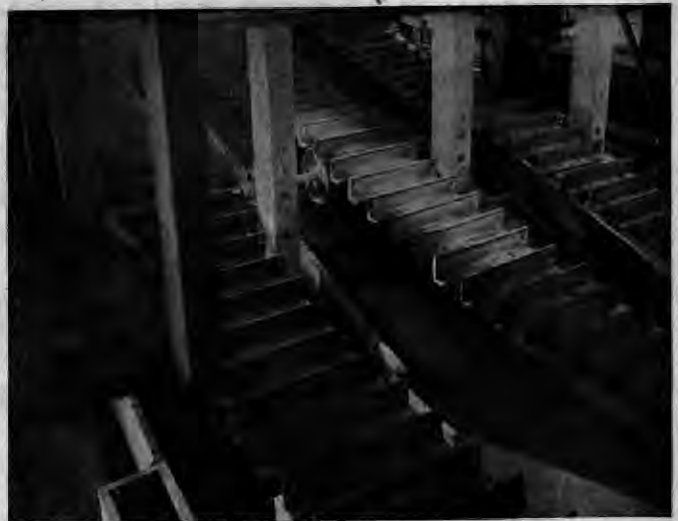
TRIPLE-BELT DRAG CLASSIFIER in the regrinding plant. The sands are delivered to the storage, or surge, bin ahead of the grinding mills. The fines after settling and thickening go direct to flotation.
