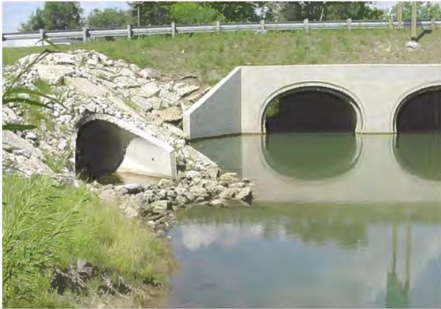
Figure 2. Culvert, riprap, and drain downstream from the intersection of Zeeb Road and Honey Creek (site 15), Washtenaw County, Mich., July 29, 2003.
