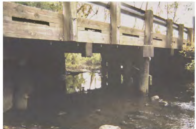
Figure 3. Bridge at site 4, Honey Creek at Pratt Rd near Ann Arbor, Mich., on September 10, 2003.
