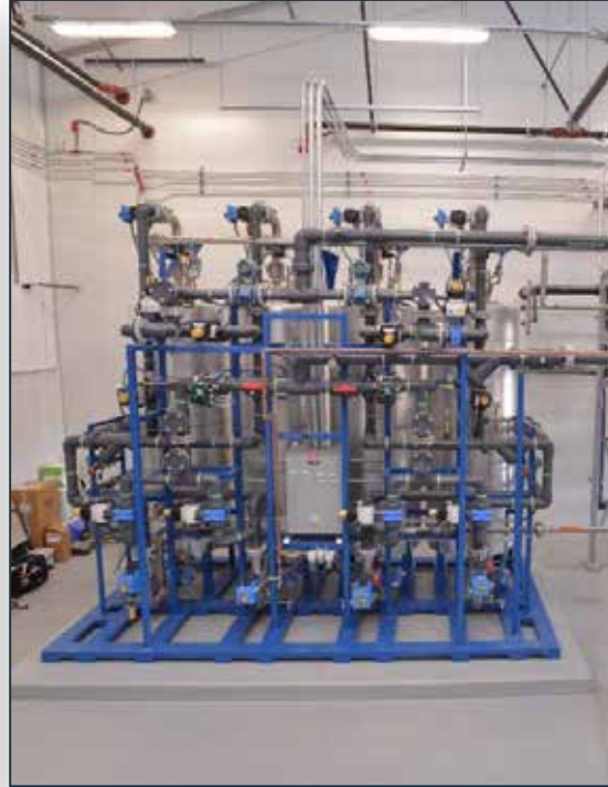
IX resin vessel skid
