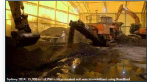
Sydney 2014: 15,000 m 3 of PAH contaminated soil was immobilized using RemBind
