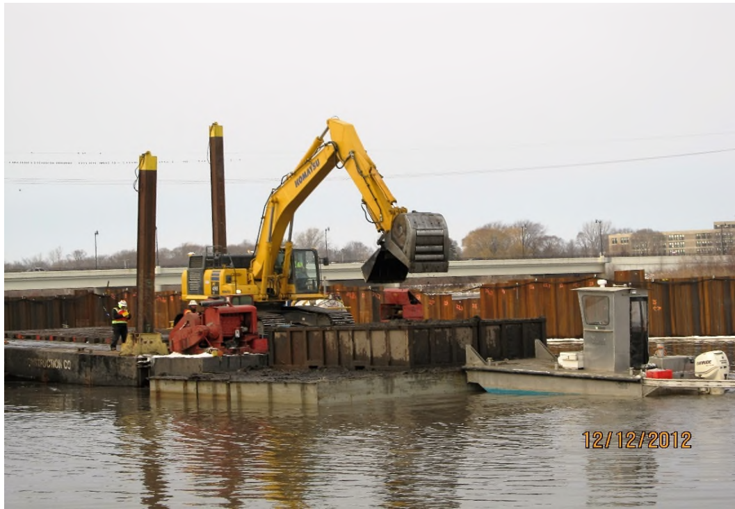
Figure 4. WPSC Former Manufactured Gas Plant Site Dredging Project 2012 (C. Bougie)
