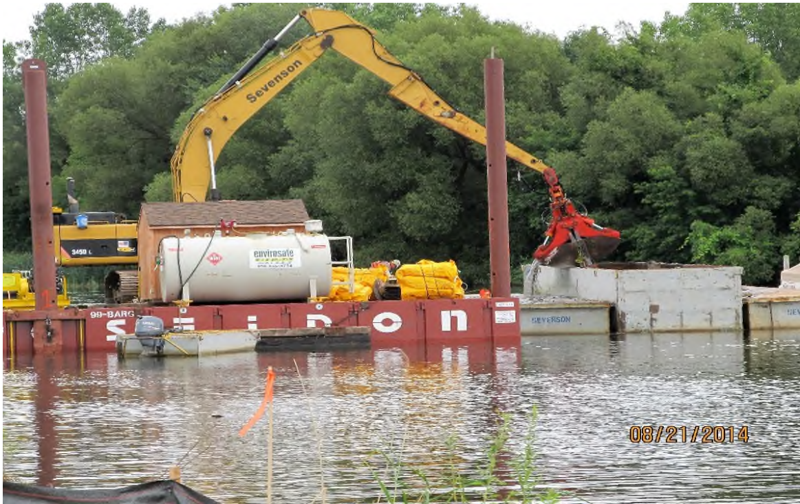
Figure 5. Menekaunee Harbor Dredging Project 2014 (C. Bougie)
