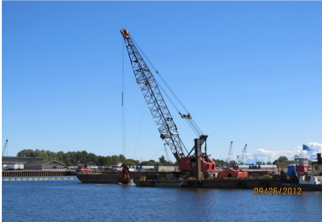
Figure 3. Ansul/Tyco Dredging Project 2012 (C. Bougie)
