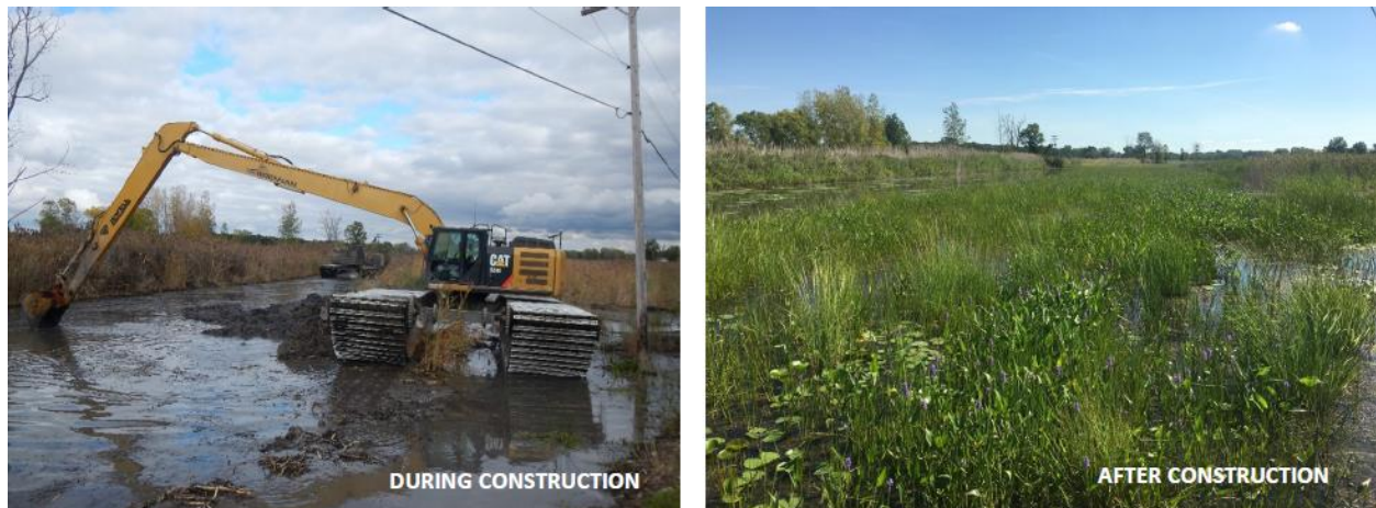
Figure 16. Before and after photographs of the Harsens Island Habitat Restoration project.
