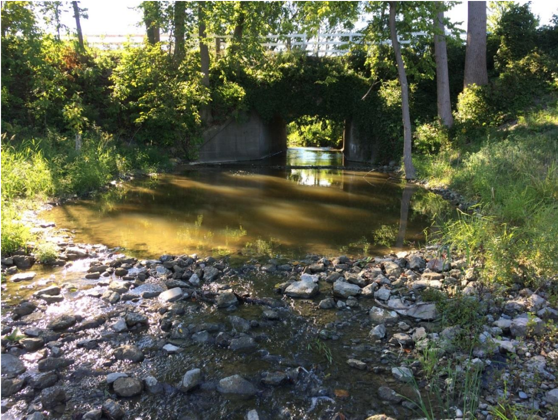
Cuttle Creek – Looking Upstream at the Formerly Perched Culvert
