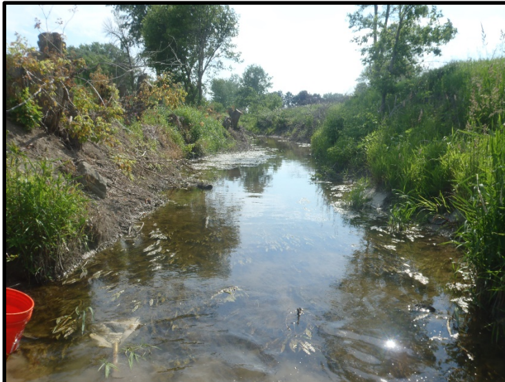
Figure 3. Figure 3. Upstream view of station S9 - Waldo Drain at Beaver Road, showing riparian removal and erosion from flashy hydrology.
