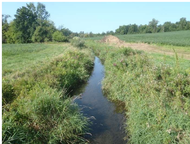
Figure 2. Perry Drain #2 upstream of Reuss Road, Shiawassee County, Michigan, September 2017.
