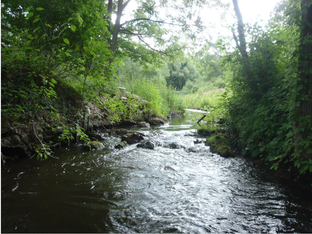
Figure 17. Dam remnants in Mason Creek downstream of Duck Lake Road, Grand Traverse County, Michigan.
