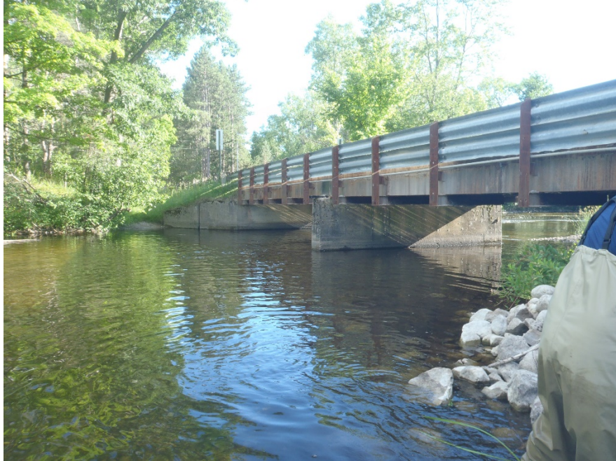
Figure 21. Betsie River upstream of Reynolds Road, Benzie County, Michigan, July 2018.
