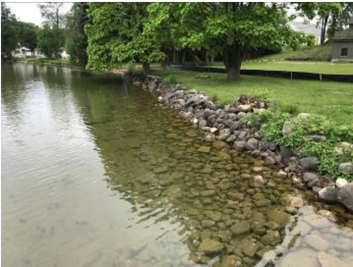
Spalding on Clam Lake Before: Maintaining turf to the water's edge. Minor erosion due to high waves overtopping existing rock revetment.
