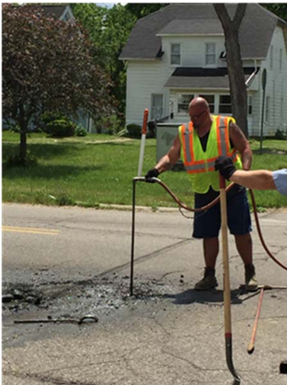
Figure 2. Jack-hammering needed to uncover paved valve on Loop #3.
