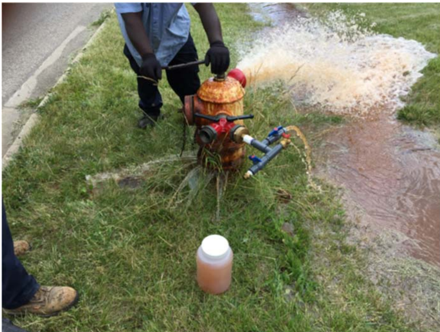
Figure 4. Hydrant for Loop #3 leaked due to broken bolts around the base flange.
