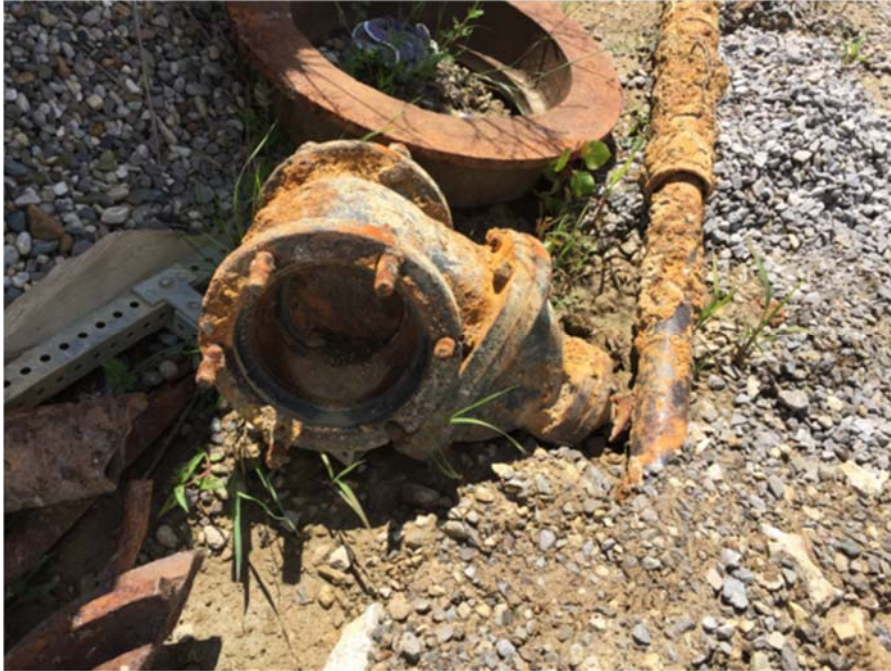
Figure 3. Example gate valve stuck in closed position (located in City boneyard).
