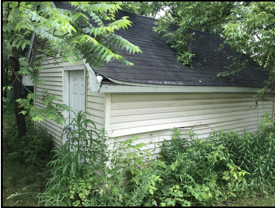
SHED EXTERIOR VIEW 53 WEST WOOD
