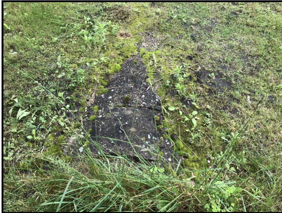
REPRESENTATIVE VIEW OF SUSPECT SEPTIC TANK OR CISTERN 53 WEST WOOD
