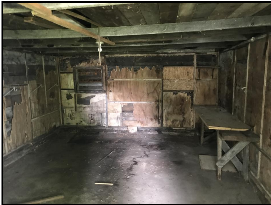
REPRESENTATIVE INTERIOR VIEW OF SHED 53 WEST WOOD
