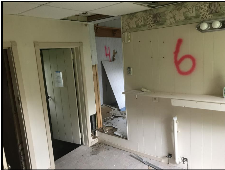
REPRESENTATIVE INTERIOR VIEW OF HOUSE 77 WEST WOOD
