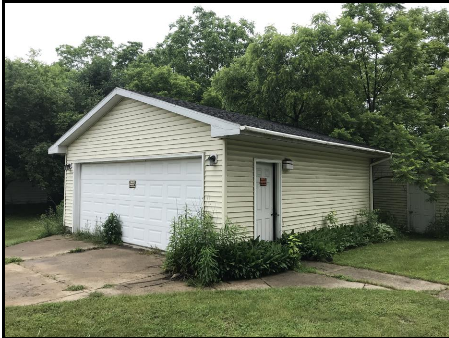
GARAGE EXTERIOR VIEW 53 WEST WOOD
