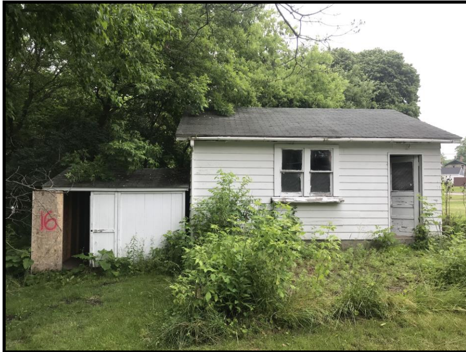
COMBINED GARAGE AND SHED EXTERIOR VIEW 77 WEST WOOD
