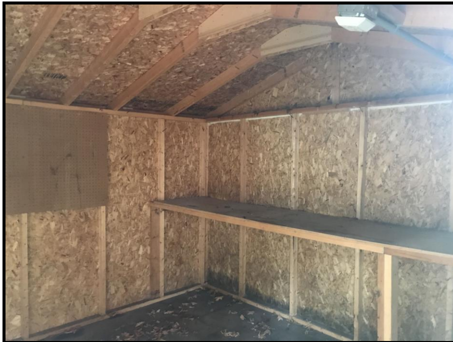
REPRESENTATIVE INTERIOR VIEW OF SHED 77 WEST WOOD
