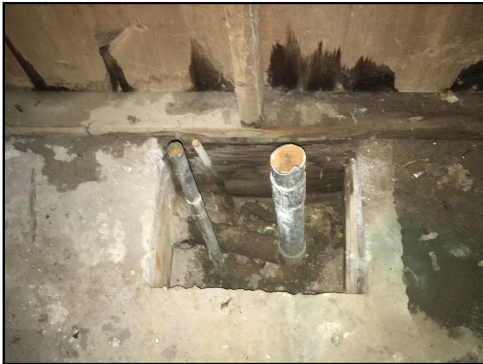
Photo 16: View of pipes that appear to have been connected to the water conditioner.
