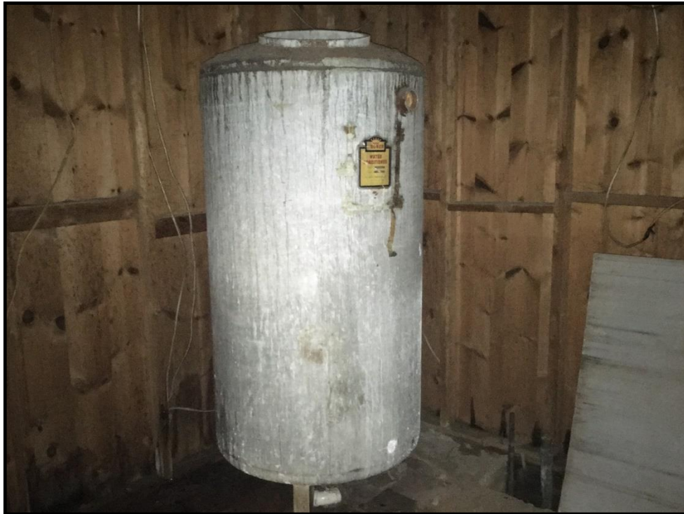
Photo 15: View of a tank labeled Water Conditioner.
