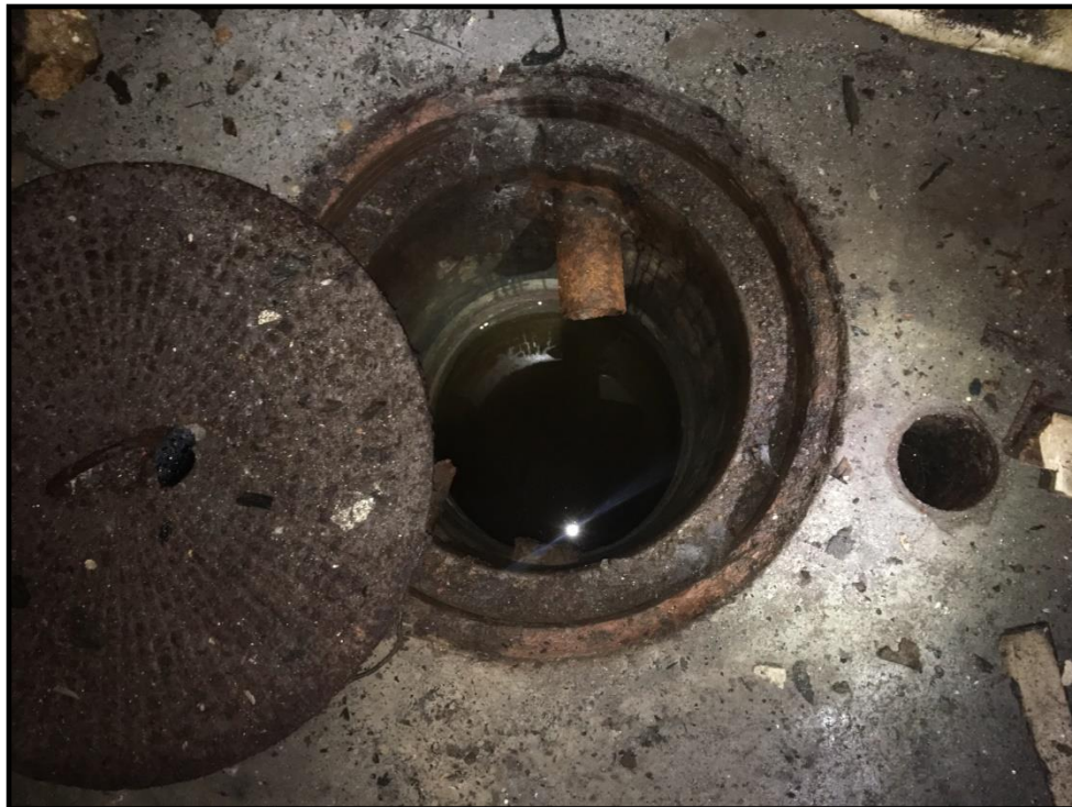
Photo 22: View of a sump and cleanout located along the southern wall inside the Property building.
