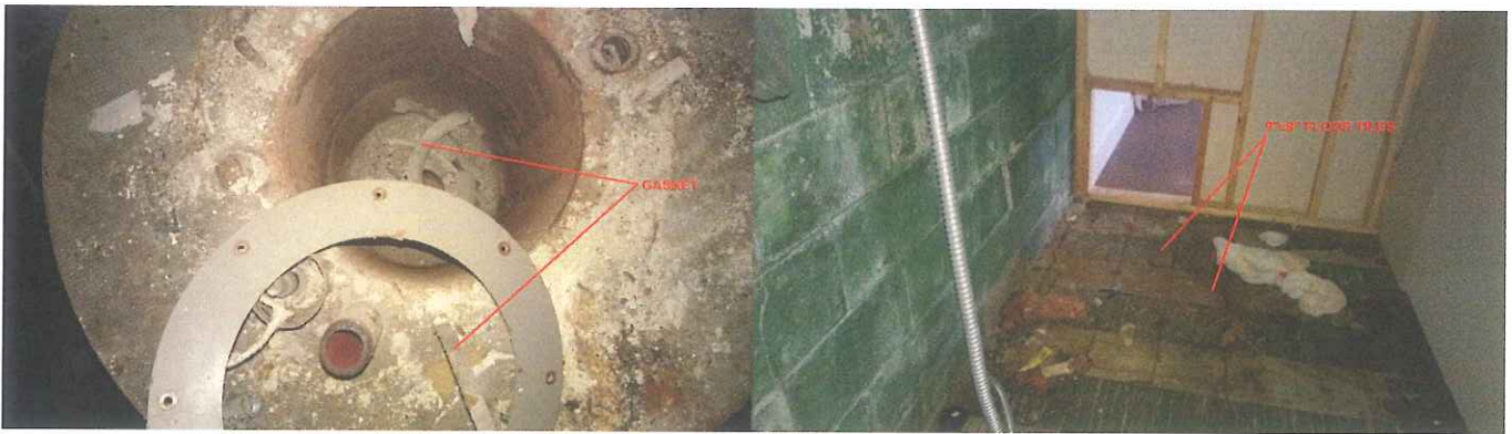
View of fibrous gasket material and two colors of 9"x9" floor tiles.
