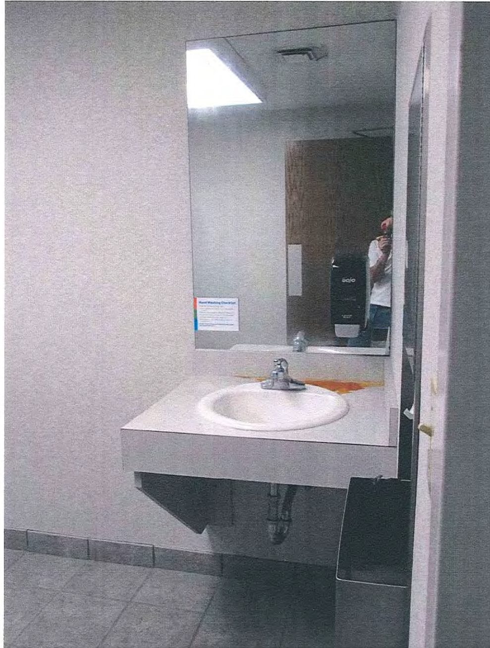
Men's Restroom - 2nd Floor
