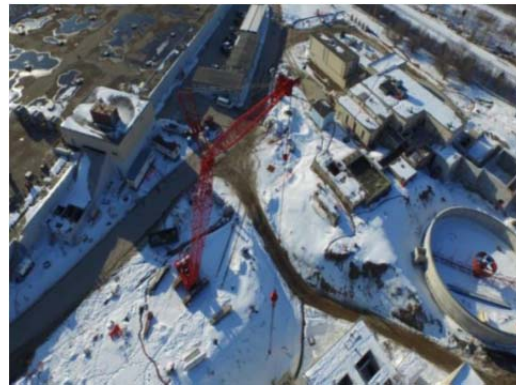
March 2015 – Aerial view of the site looking Northwest.
