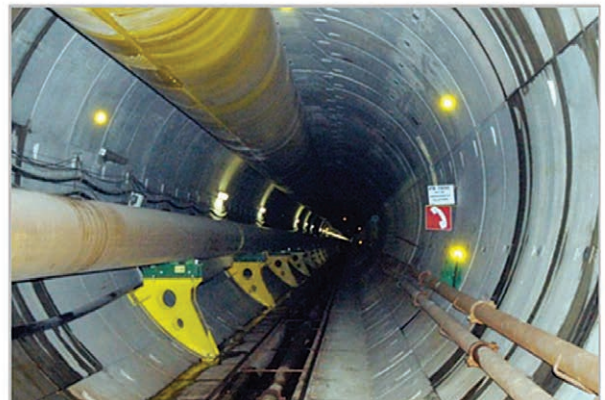
Figure 8: The GASTAU Tunnel (below), which runs below a state park in Brazil, is a 3.2-mile open and accessible tunnel with a 28-inch diameter high-pressure gas pipeline leading to a refinery. The tunnel was excavated using a TBM and a pre-cast concrete lining.
