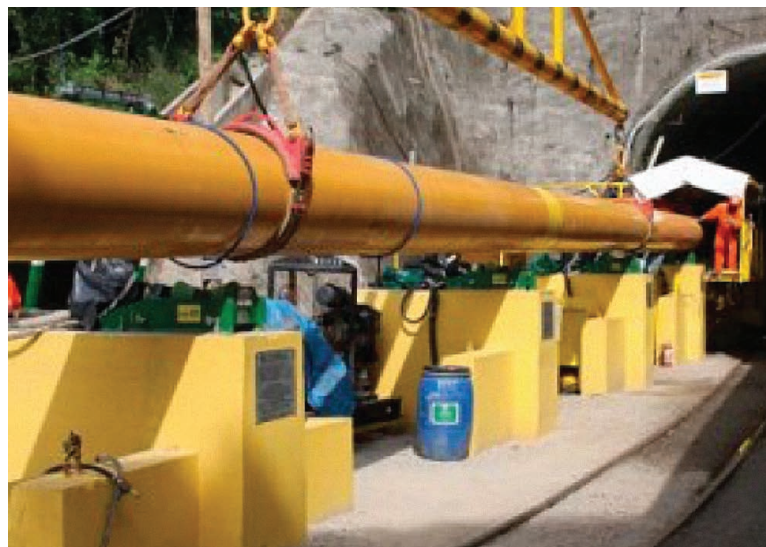
Figure 17: Section of welded pipe string being lifted onto rollers in preparation for being installed in tunnel.
