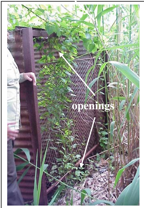
Figure 2. Structure of weir at north end of Grassy Island, Detroit River, Michigan.
