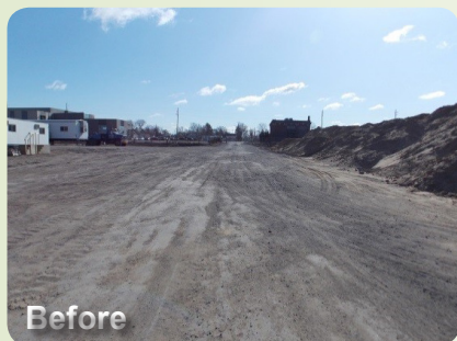
East Main Street construction (facing east)
