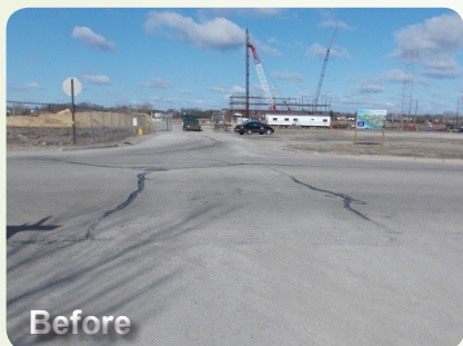
East Main Street construction (facing west)
