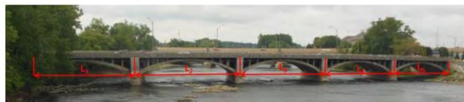
Figure 5.13.07 Horizontal Length along the Traveled Way Must Be Used for Arches
