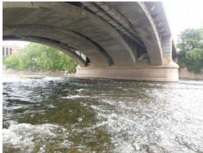
Figure 5.13.06 Open Spandrel Concrete Arch with Multiple Ribs
