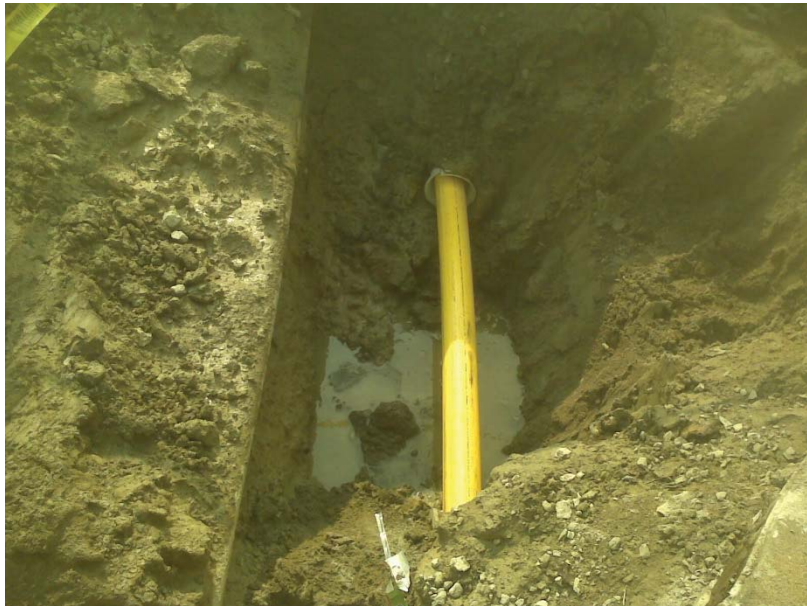
Figure 10: 4" MDP Gas Main Inserted into Existing 6" Cast Iron Main
