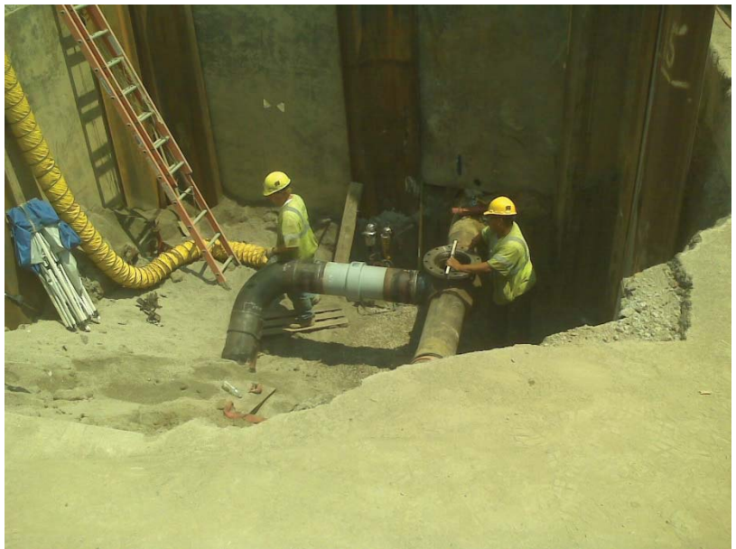
Figure 9: 12" High Pressure Gas Main in Open Excavation
