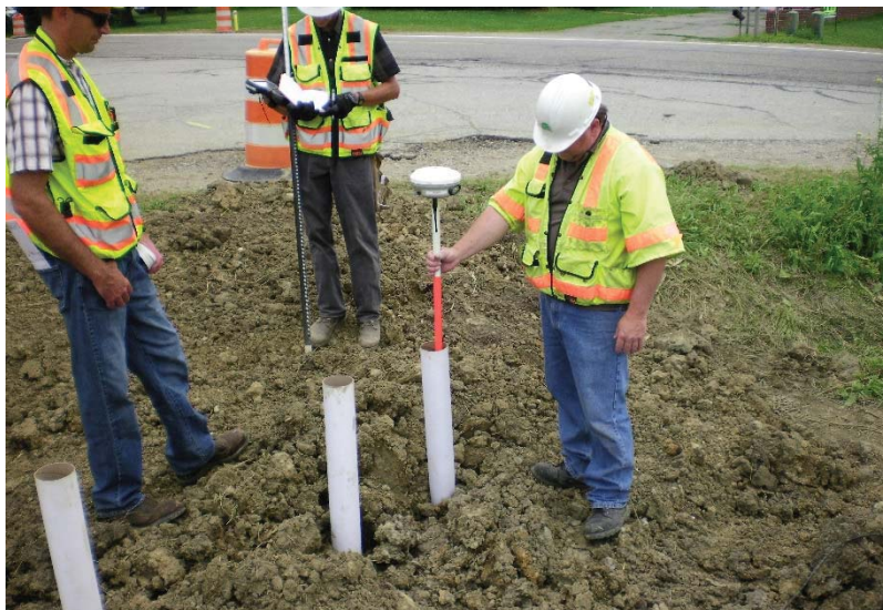
Figure 3: Surveying Utility inside Cardboard Tube
