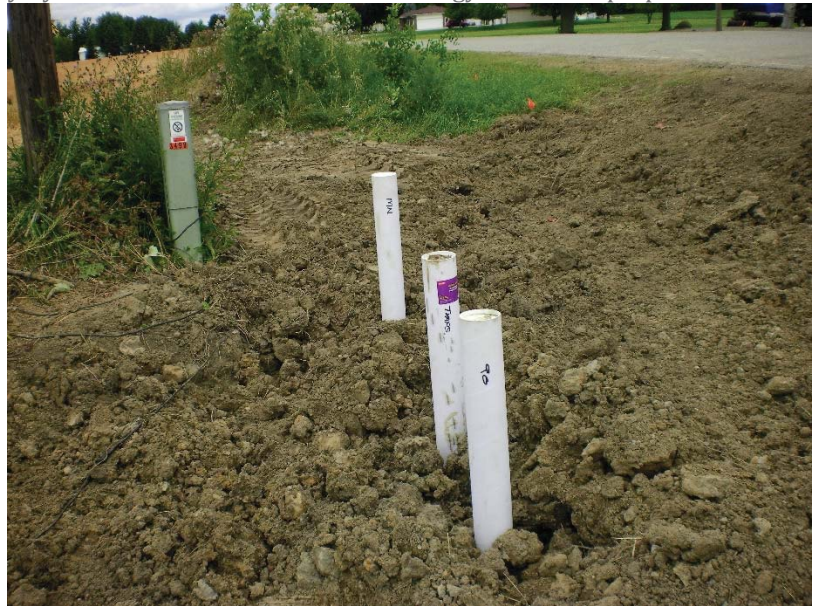
Figure 2: Cardboard Tubes Placed over Gas Main
