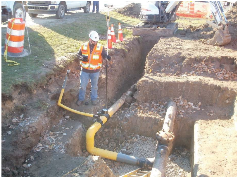
Figure 6: Surveyor Recording a GPS Observation on Gas Main in Open Cut Section
