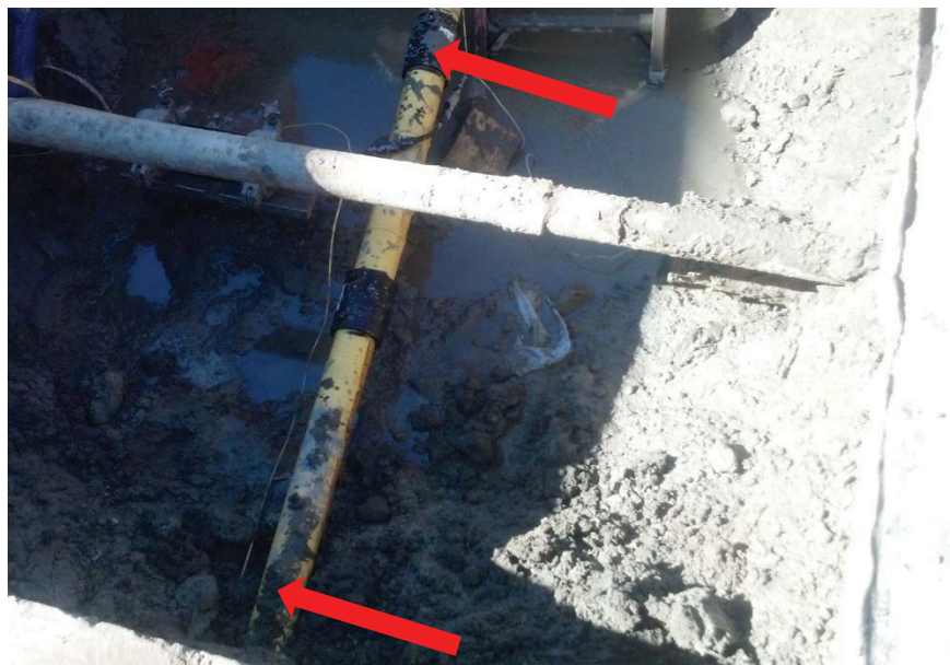
Figure 11: Installation Pit for Insertion Method. Survey Observation Locations Identified
