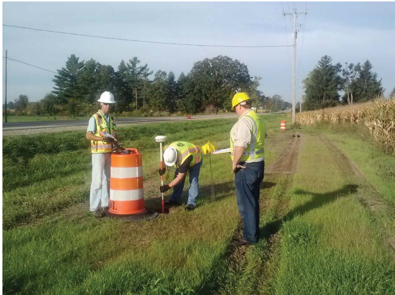
Figure 5: Survey Crew Obtaining Positional Data on Exposed Utility
