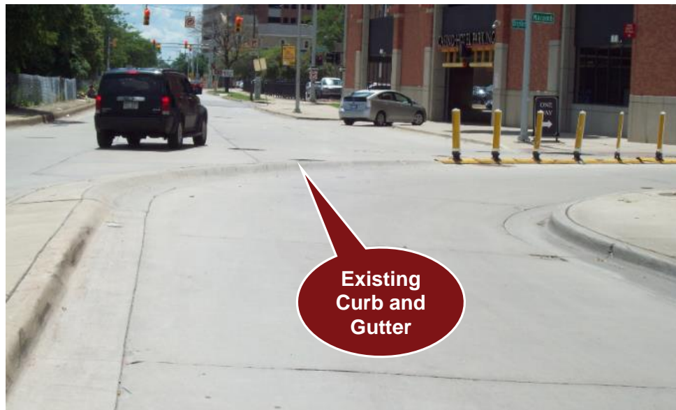
Figure 4.14.1 – Curb on SB Chrysler Drive at Macomb St
