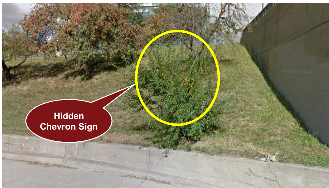
Figure 4.15.1 – Vegetation Obscuring Sign on NB I-375
