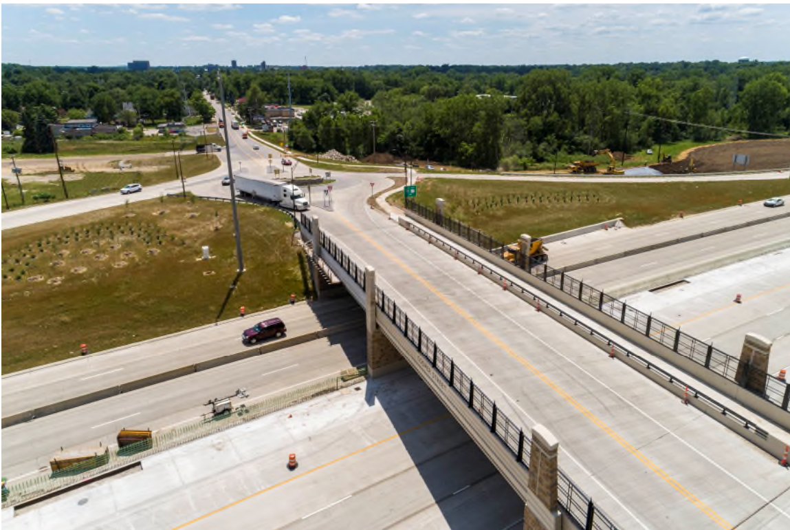
Figure 1: Cooper Street Interchange over I-94 in Jackson, MI
