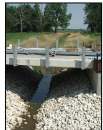
Figure 2: Slab bridge
