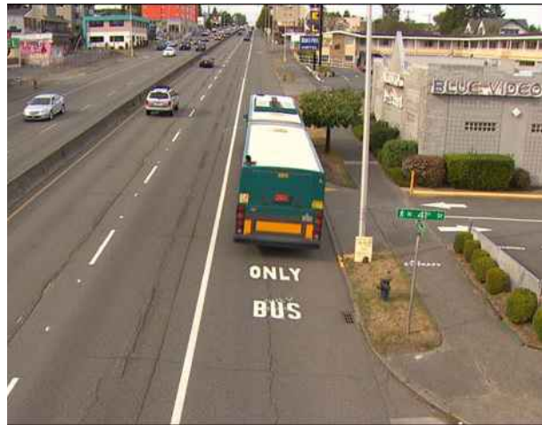
The Denver Region has implemented low cost dedicated bus lanes using paint and signage that preserve space for transit until a larger investment can be made.
