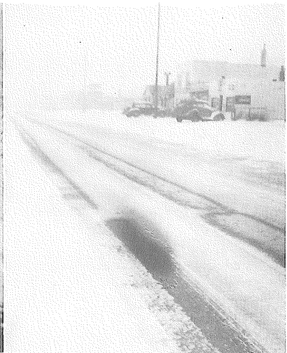
▲ FIGURE 8. VIEW OF HEATED BIT- UMINOUS SECTION ( 3-17-50 ) J.A.W.
