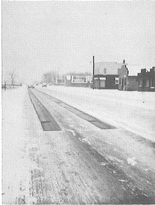
▲ FIGURE 1. BITUMINOUS SECTION ( 1 - 6 - 50 ) HEATED AREAS CLEAR
