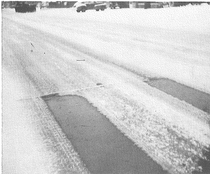
▲ FIGURE 3. CONCRETE SECTION ( 1 - 6 - 50 ) ICY CONDITION AT END OF SECTION
