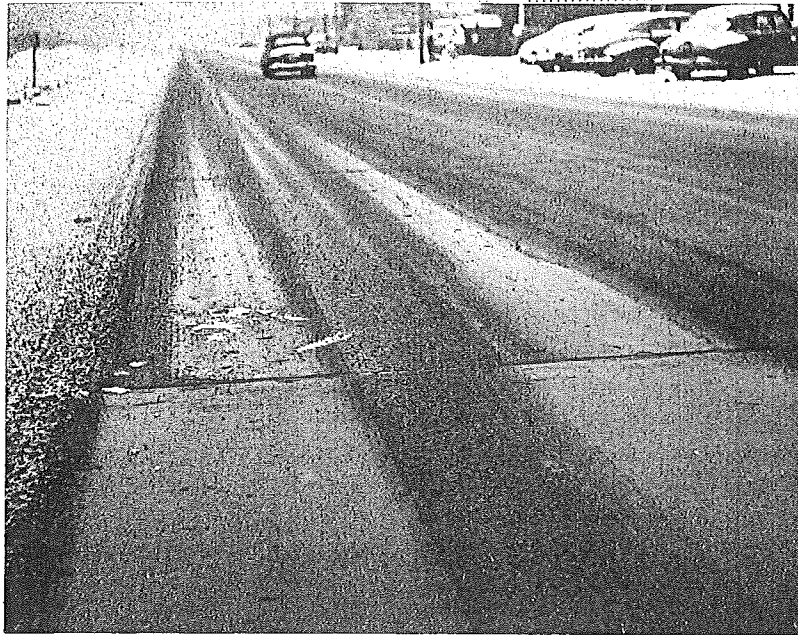
FIGURE 3. VIEW SHOWING TYPICAL ICE BUILD-UP ADJACENT TO HEATED AREAS. RIDGES ON BITUMINOUS SECTION - 2 INCHES HIGH. STORM 1/15/51
