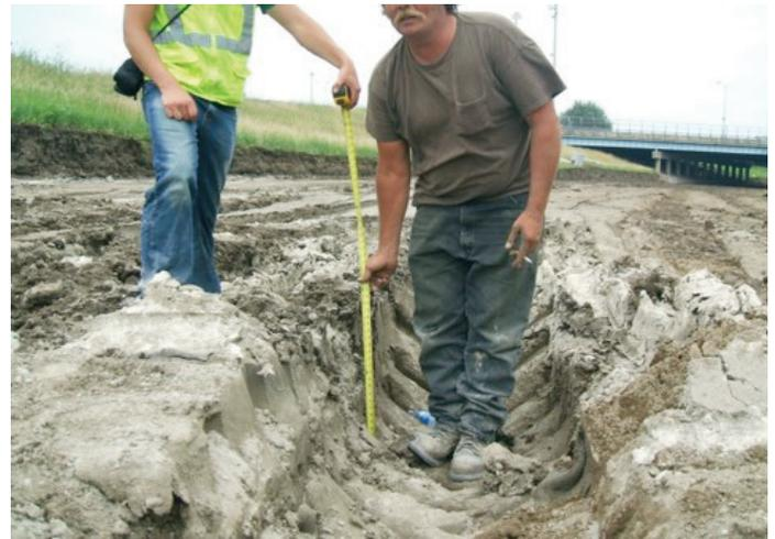
Weak subgrade soils may lead to significant failures under construction traffic loading.
