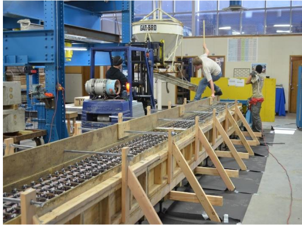
Figure 4.3-8 Placing concrete in the formwork
