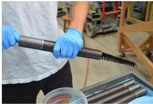
(c) Cleaning the socket
