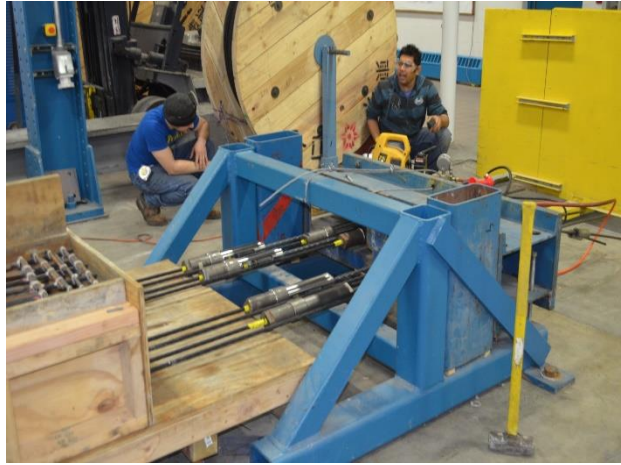
Figure 4.3-7 Applying prestressing force using a hydraulic pump
