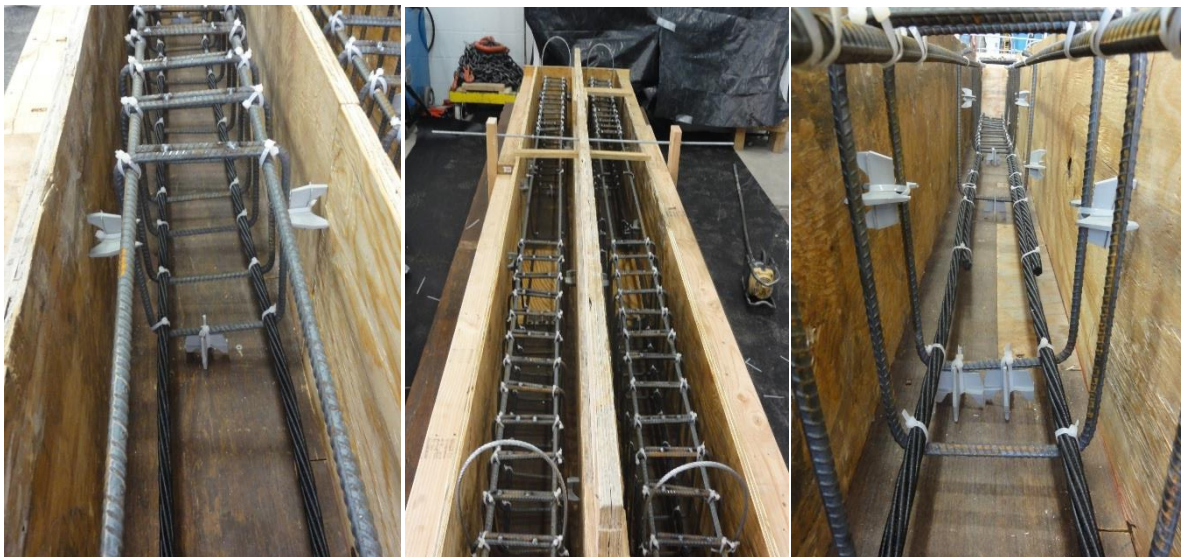
Figure 7.3-5 Placing the reinforcement cages in the formwork
