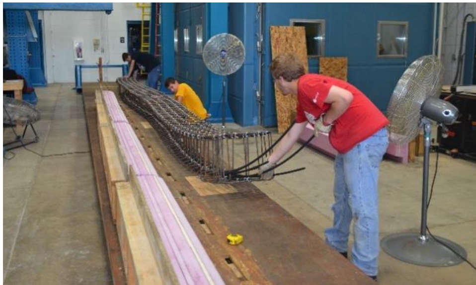
Figure 8.2-9 Bottom prestressing installation
