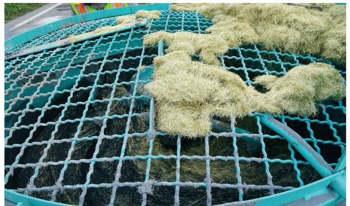
Near the end of the MI-UHPC mixing process, crews add steel fibers through a grate over the mixing barrel.
