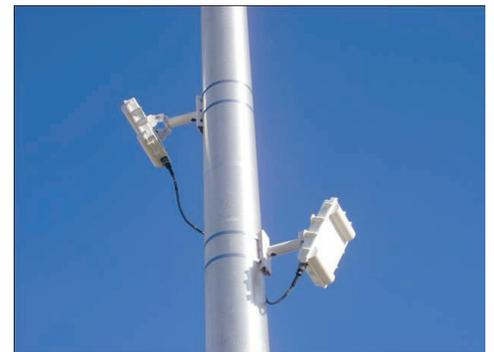
Researchers proposed adding nonintrusive MVDS sensors (shown here on roadside poles) to MDOT's traffic monitoring network to improve coverage while reducing installation and maintenance costs.
