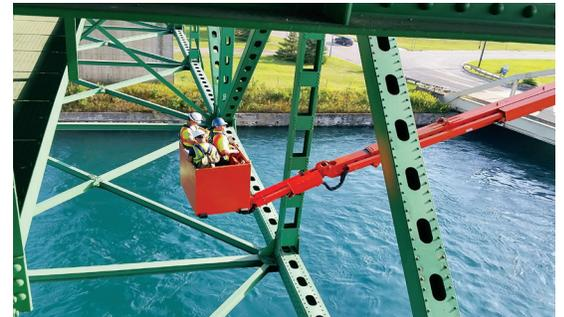
Large, complex bridges require inspection methods such as the use of underbridge inspection units (UBIUs) that reach from above deck to below.
