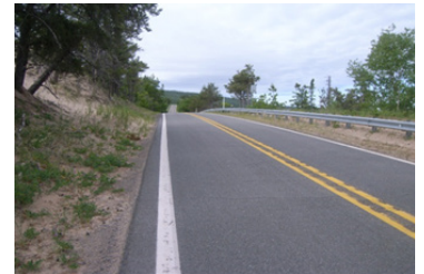
M-26 near Great Sand Bay between Eagle River & Copper Harbor has no paved shoulders (photo courtesy of WUPPDR)
