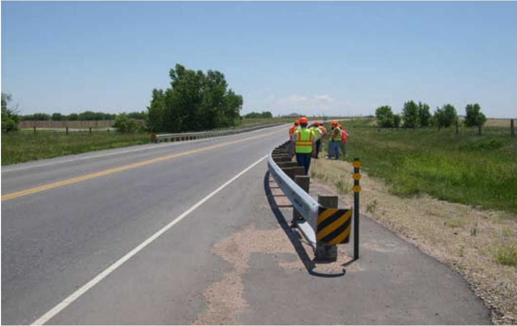
Figure 22. Guardrail terminal and pavement in Colorado.
