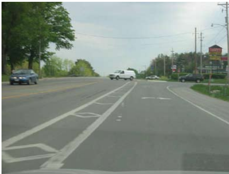
Figure 6. Addition of turning lane in Iowa. (Source: Courtesy of IADOT)
