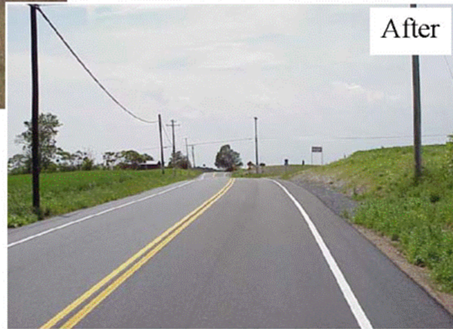
Figure 8. After resurfacing and realignment to improve intersection sight distance in New York. (Source: Courtesy of NYSDOT)
