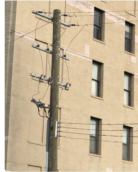
After Hardening Work
