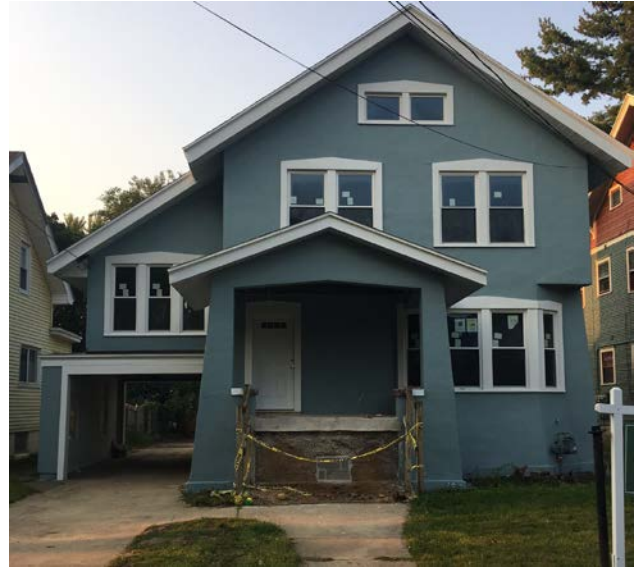
GR City HOME – Grand Rapids - Rehab Completed in the Fall of 2017
