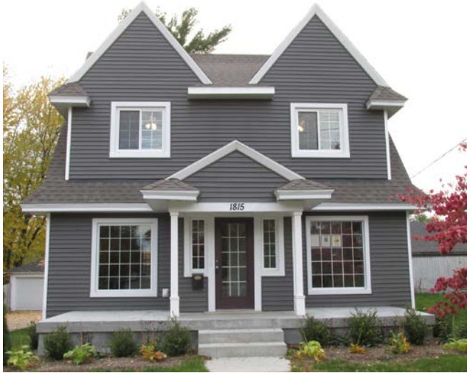
GR City HOME – Grand Rapids - Rehab Completed in 2013
