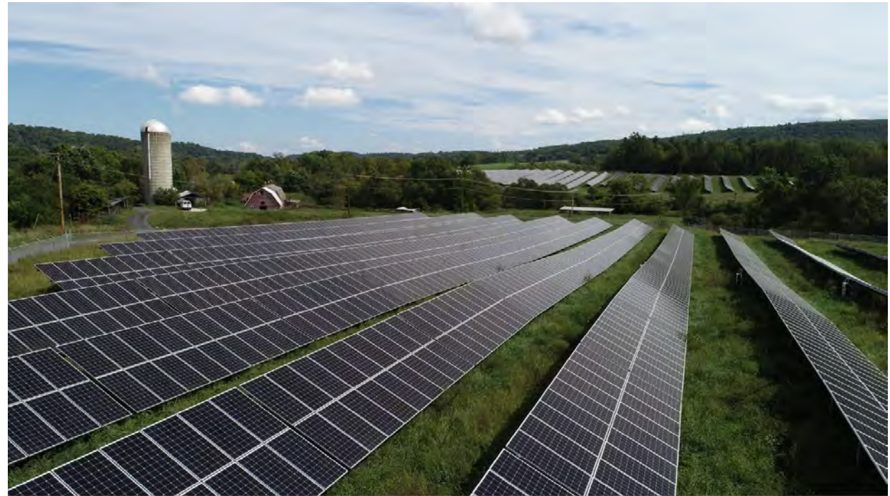
Source: Borrego Solar, Buckley Solar Project (NY)
