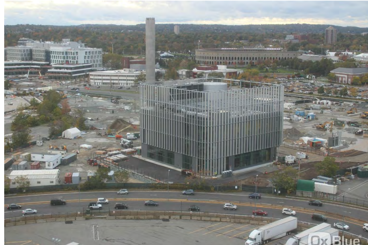
New District Energy Facility 2019 – 5.2 MW Allston Campus Development
