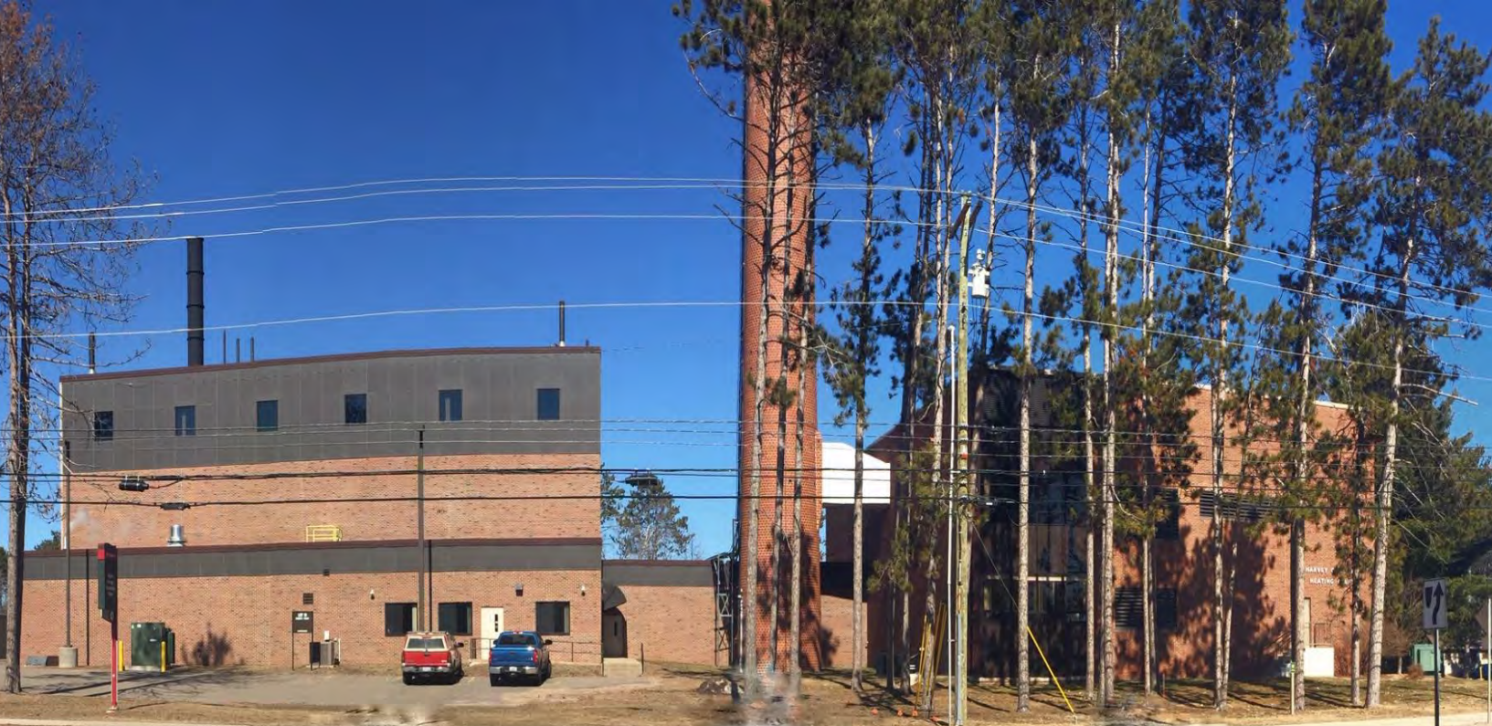
CHP Plant Addition
