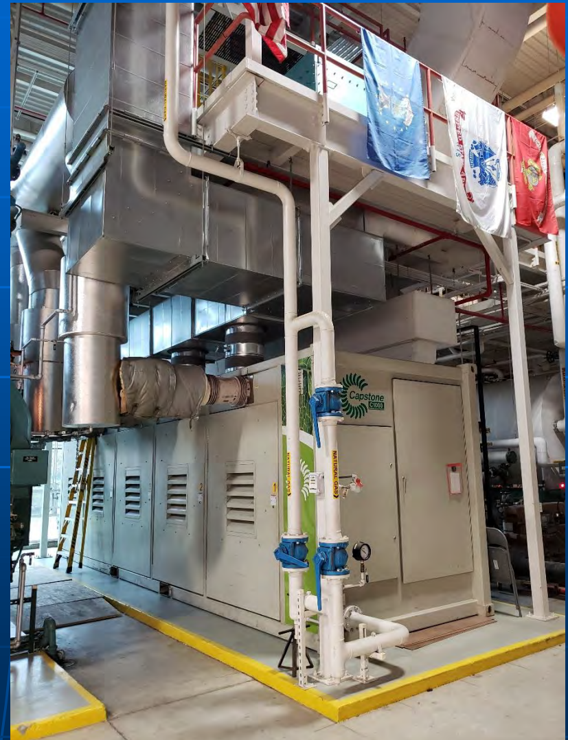
Natural Gas Fired Turbines
