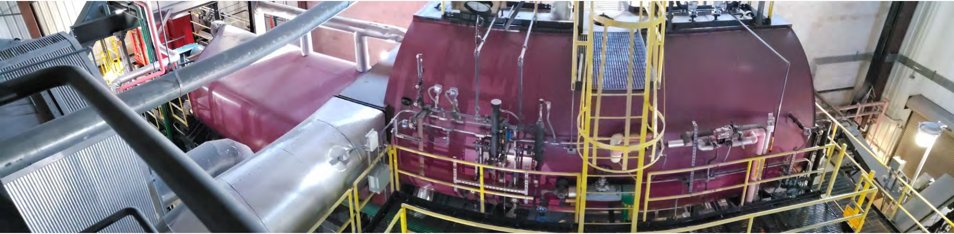
Boiler Water Tube Section & Economizer
