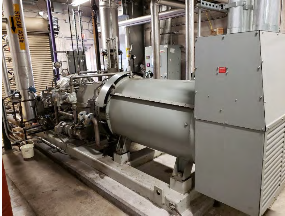
Backpressure Steam Turbine Generator
