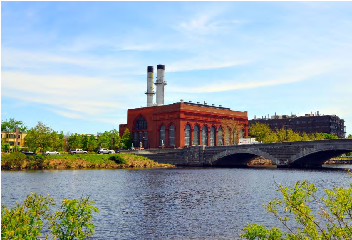
Blackstone (orig 1902) – 5 MW backpressure turbine; 8 MW combustion turbine in 2015
