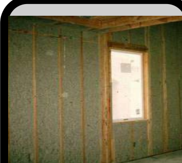
Insulation Installation
