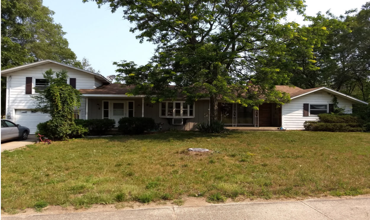
Grant# HDF-2019-580-NEP, Housing Enhancement, Before 831 Adda St.
