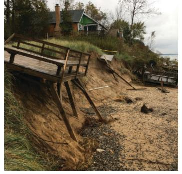
Erosion has led to the collapse of two decks along Lake Michigan, scattering debris along the shore. (Photo courtesy of EGLE)
